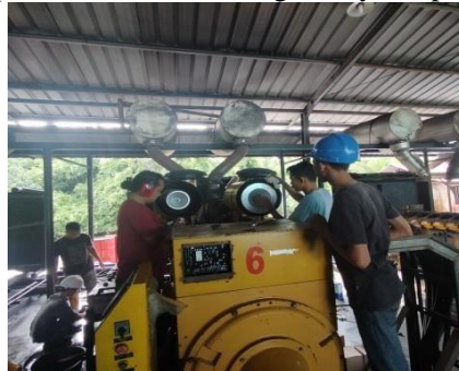
Gambar 2.21 Kegiatan penggantian filter (Sumber: PT. Megapower Makmur Tbk, 2023)
