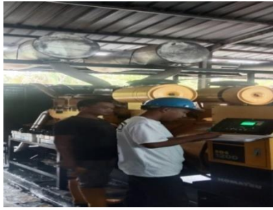
Gambar 2.2 Kegiatan monitoring KWh ( sumber : PT. Megapower Makmur Tbk, 2023)
