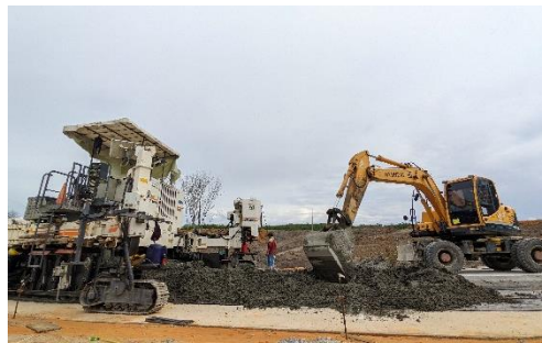
Gambar 4.10 Penghamparan beton dibantu wheel escavator
