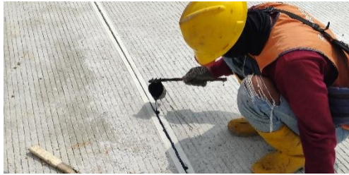
Gambar 4.17 Pekerjaan joint sealer
