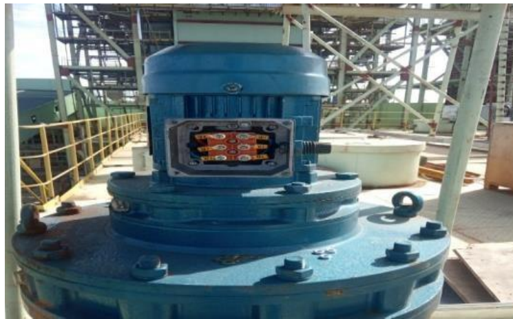
Gambar 3.11 Motor Rapping Sumber: Google Searching.com
