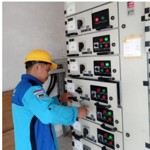
Gambar 2. 30 Proses penormalan Braker Motor Intermediate pump (Sumber : Dokumentasi 2023)
