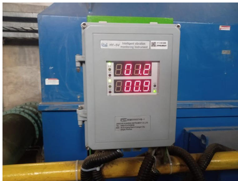
Gambar 3. 28 Data Vibrasi Motor CWP 2B Intelligent Vibration Monitoring Instrument (Sumber: Dokumentasi 2023)
