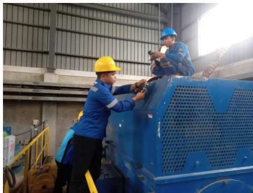
Gambar 2. 34 Proses Change over Cooler Motor CWP (Sumber : Dokumentasi 2023)
