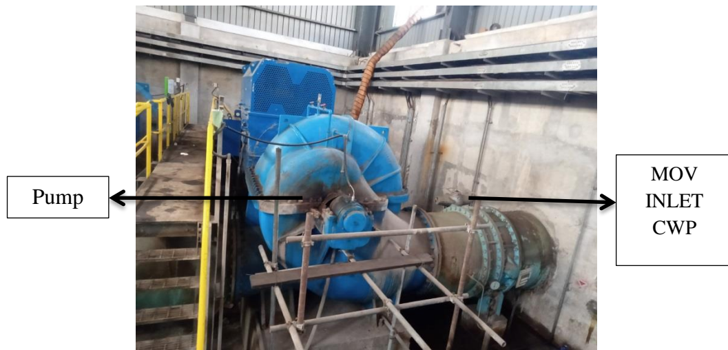
Gambar 3. 2 Circulating Water Pump (CWP)
