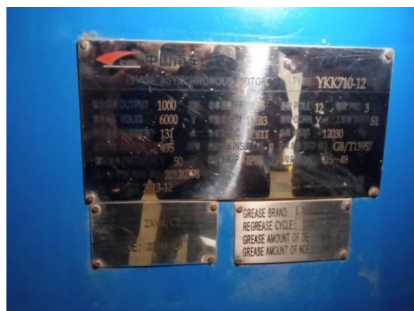
Gambar 3. 3 Nameplate Motor Circulating Water Pump (CWP)
