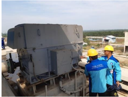
Gambar 2. 7 Proses Regreasing Colling Tower (Sumber : Dokumentasi 2023)
