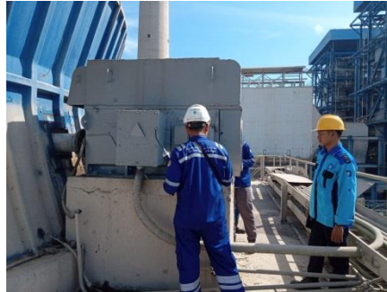
Gambar 2. 5 Proses Regreasing Cooling Tower (Sumber : Dokumentasi 2023)
