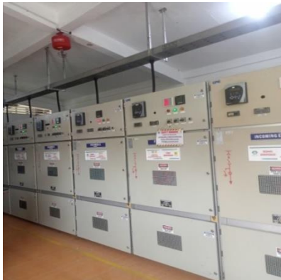
Gambar 2. 19 Pengecekan evidence beban feeder Sumber: PT. Adra Gemilang. 2023
