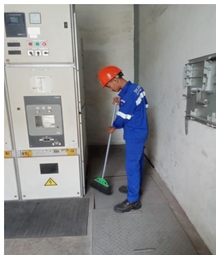
Gambar 2. 2 Cleaning trafo room
