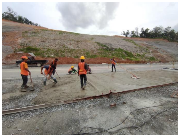
Gambar 4.1 Pekerjaan Lean Concrete
