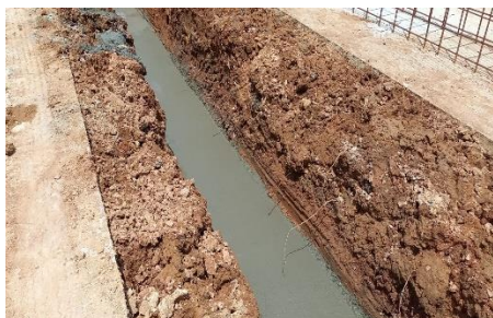
Gambar 4. 15 proses pengecoran LC
