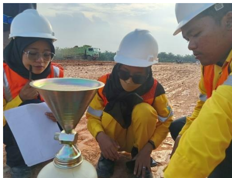
Gambar 3. 24 proses pengujian sane cone
