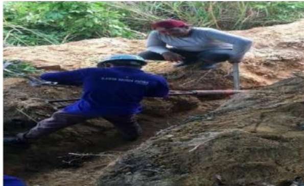
Gambar 2.15 Jointing Kabel Sumber: Dokumentasi, 2022
