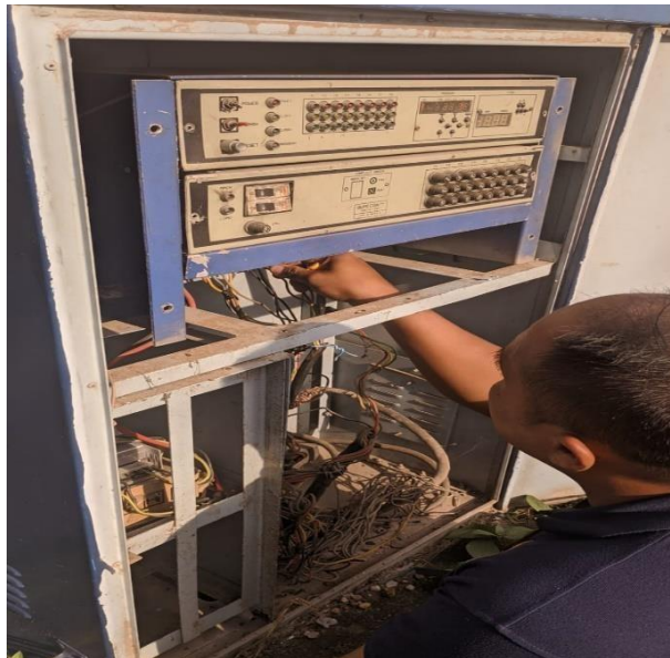
Gambar 3.4 Pengecekan Kendai Traffic Light
