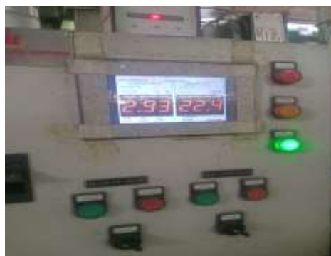
Gambar 2. 21 Monitoring Steam di Turbin Sumber Dokumentasi 2023
