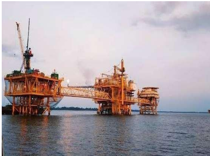
Gambar 1.3 Well Lalang Platform (Sumber : PT.Imbang Tata Alam 2022)
