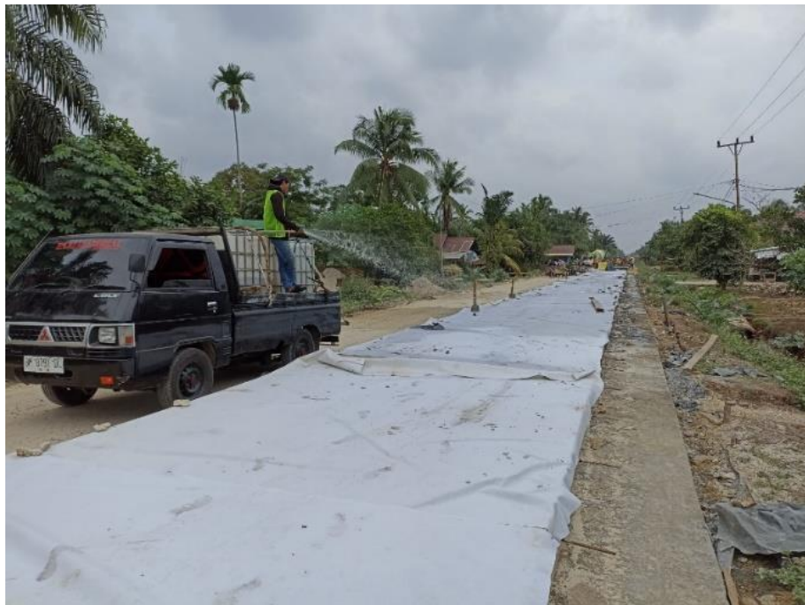
Gambar 27 Proses Curing
