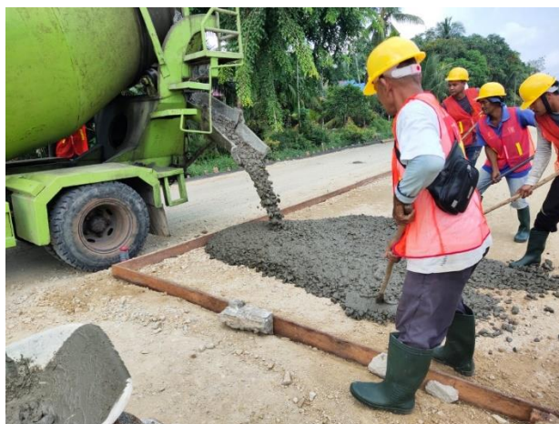
Gambar 21 Pengecoran Lantai Kerja (Lean Concrete)
