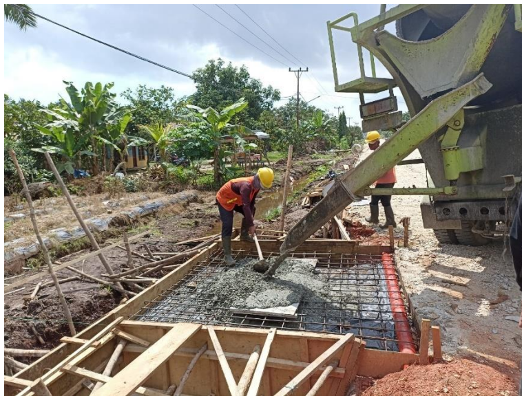
Gambar 12 Pengecoran box culvert
