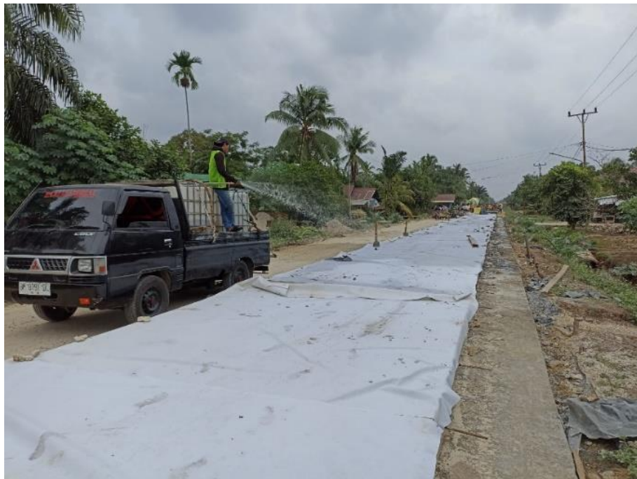
Gambar 27 Proses Curing
