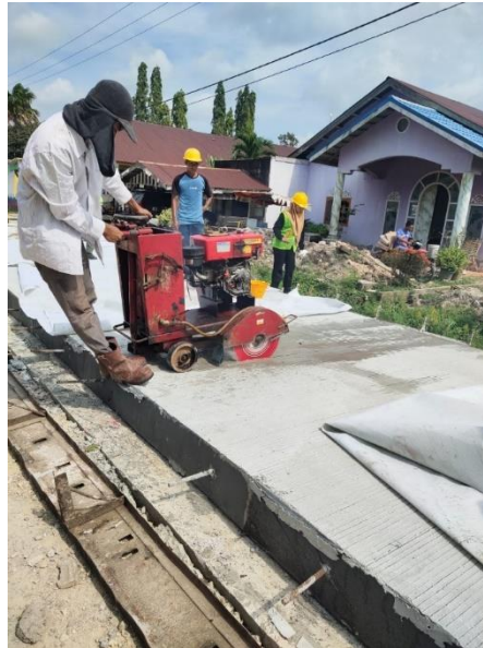
Gambar 28 Proses Cutting
