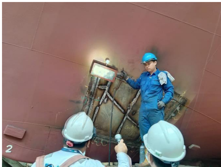
Gambar 2.5 Uji Vakum test
