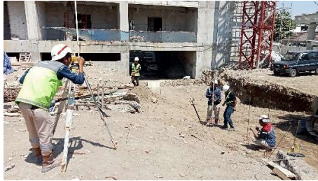
Gambar 3. 37 Marking Bouplank lanscape
