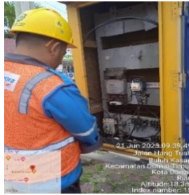
Gambar.2.13. Pengantian MCB (Sumber PT.Haleyora Power,2023)
