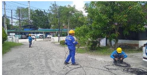
Gambar.2.2 pengantian kabel SR (Sumber PT.Haleyora Power,2023)
