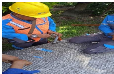
Gambar.2.44. Pengantian fuse link (Sumber PT.Haleyora Power,2023)
