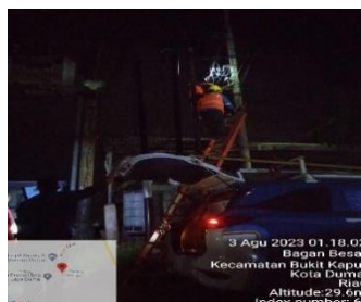
Gambar.2.41. Penyambungan incoming (Sumber PT.Haleyora Power,2023)
