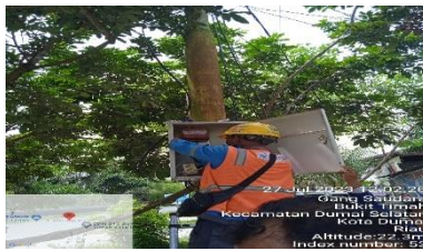
Gambar.2.35. Pegantian KWH (Sumber PT.Haleyora Power,2023)
