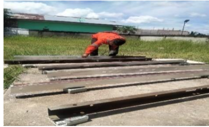
Gambar.2.7.Memperbaiki traves. (Sumber PT.Haleyora Power,2023)
