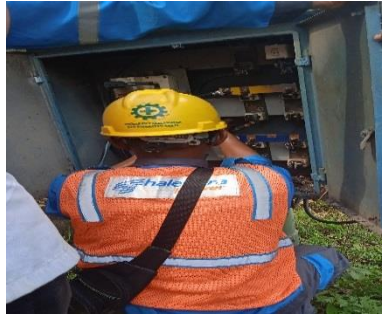
Gambar.2.43. menggantikan pin copper (Sumber PT.Haleyora Power,2023)
