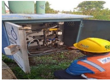
Gambar.2.26 Memasang NH fuse (Sumber PT.Haleyora Power,2023)
