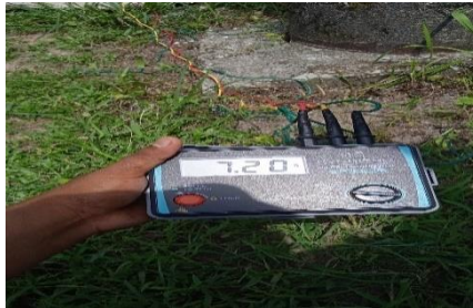
Gambar.2.42. Pengecekan Gronding LA (Sumber PT.Haleyora Power,2023)
