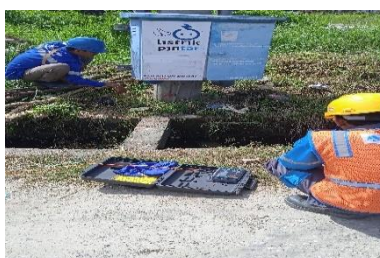
Gambar.2.19.Pengukuran tegangan grounding (Sumber PT.Haleyora Power,2023)
