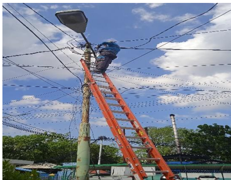
Gambar 3.2 Penggantian Pierching (Sumber PT.Haleyora Power,2023)
