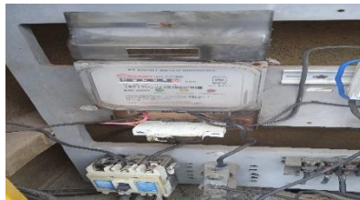
Gambar.2.25 Mengatasi gangguan KWH (Sumber PT.Haleyora Power,2023)
