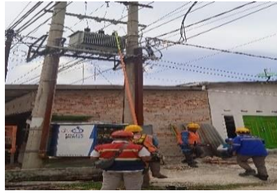
Gambar.2.11. Pemasangan grounding trafo (Sumber PT.Haleyora Power,2023)
