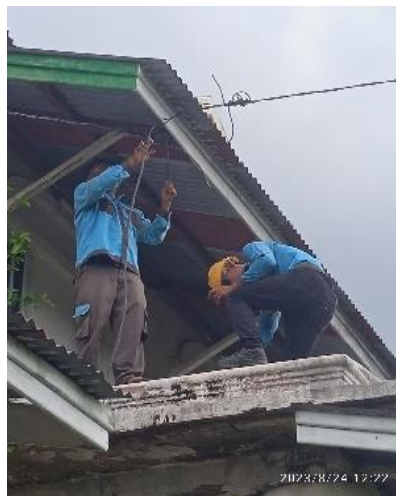
Gambar 2. 51 Mengatasi Lost contact
