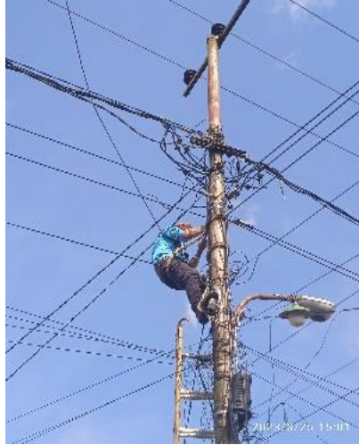
Gambar 2. 52 Mengatasi Lost contact
