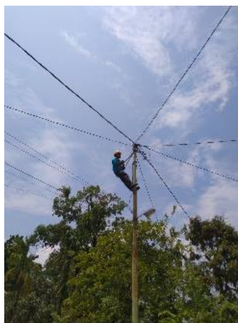
Gambar 2. 53 Mengatasi Lost contact
