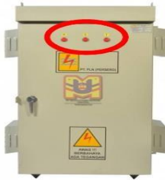
Gambar 3. 7 Lampu indikator PHB TR
