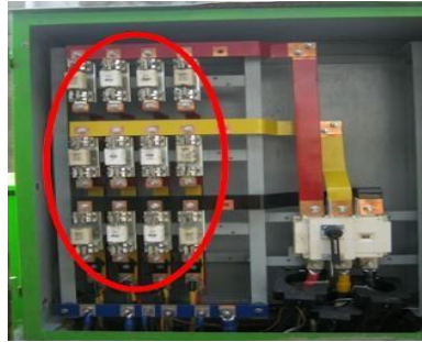
Gambar 3. 4 NH /NT Fuse PHB TR
