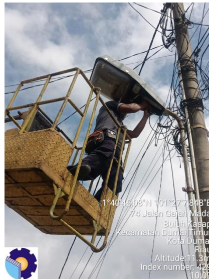
Gambar 2.43 Memasang lampu LED Hori
