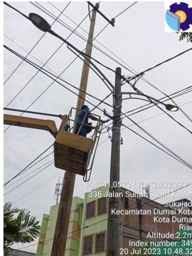
Gambar 2. 32 Memasang suspantion
