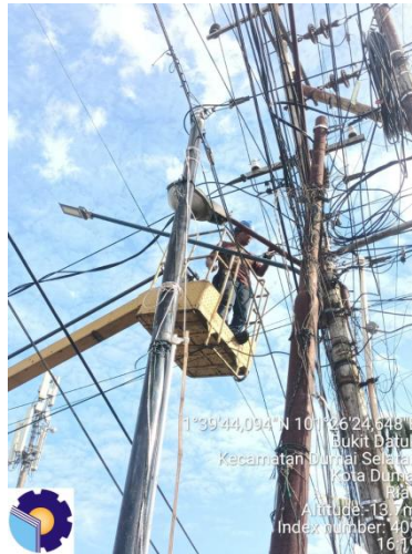
Gambar 2. 40 Memasang lampu LED
