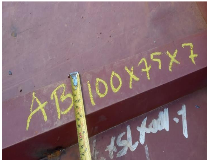
Gambar 2.6 Fit-Up Angle Bar
