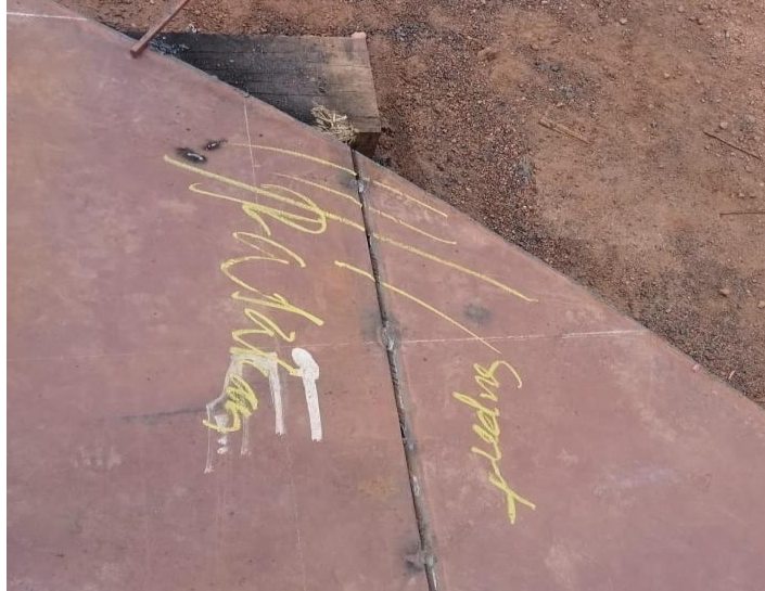
Gambar 2.49 Fit-Up Raised Deck
