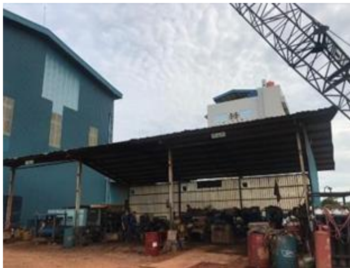
Gambar 1.11 Workshop Mechanical & Electrical
