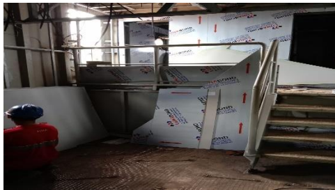
Gambar 2.75 Pemasangan Aluminium ( Outfitting )
