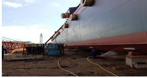
Gambar 2.41 Persiapan Launching pengisian balon air bag system
