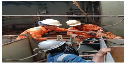
Gambar 2.47 Pemasangan Plate Engine Girder
