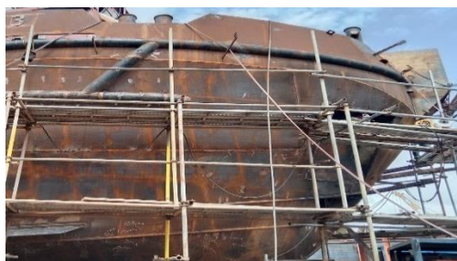
Gambar 2.34 Body Fore Peak dan Chain Locker
