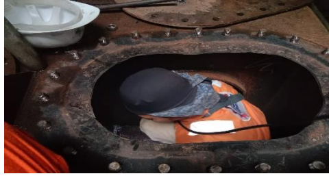
Gambar 2.62 Pengecekan Kebocoran Tangki Kapal Tug Boat
