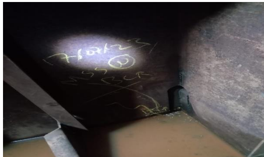
Gambar 2.27 Pengecekan Kebocoran Tangki Kapal Khususnya Bulk Head
