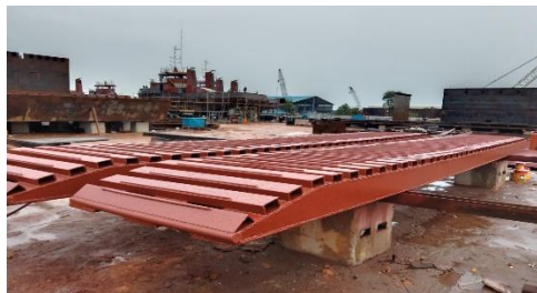
Gambar 2.64 Blasting dan Painting Rampdoor
