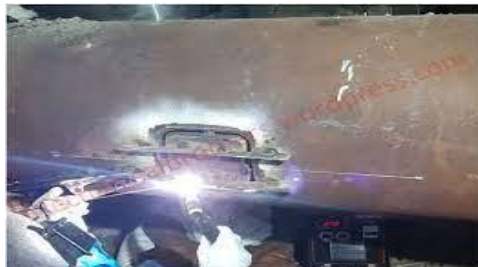
Gambar 2.13 Insert plate
