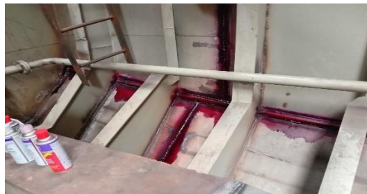
Gambar 2.99 Penetran Test bagian Side Sheel, Roundbar, Chine, dan Engine Girder
