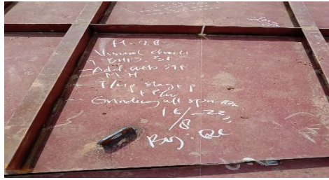
Gambar 2.94 Inspeksi Visual Fitt Up dan Welding Main Deck Kapal Tug Boat
