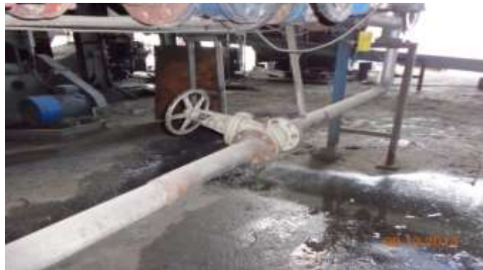
Gambar 3.142. Modulating control valve
