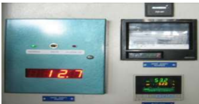
Gambar 3.14 Water level control
