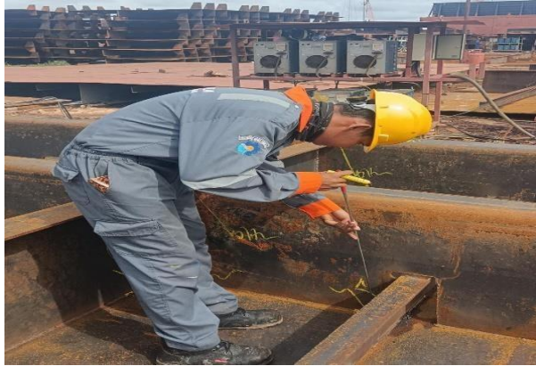
Gambar 2. 18 Inspect welding terhadap main deck
