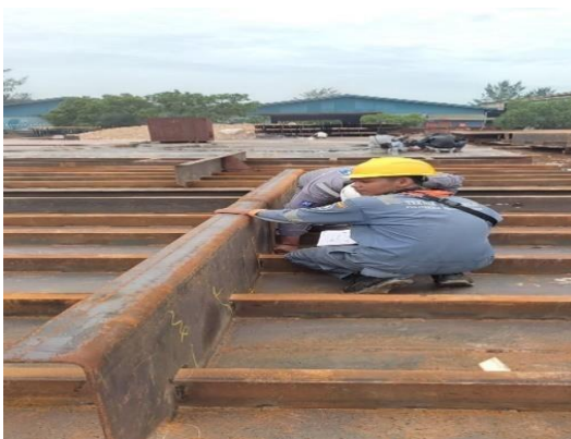
Gambar 2. 7 Inspect welding terhadap Transverse Bulkhead
