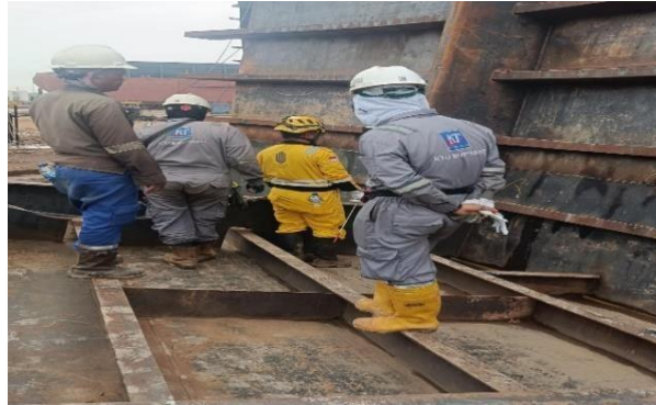
Gambar 2.20 inspec welding Bersama Owner
