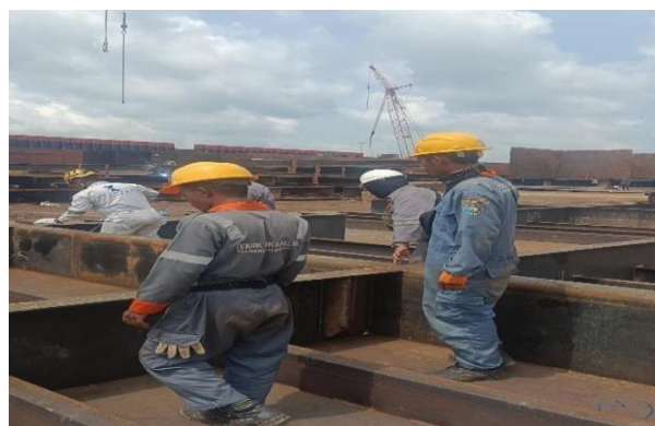
Gambar 2. 29 inspect welding Bersama Owner
