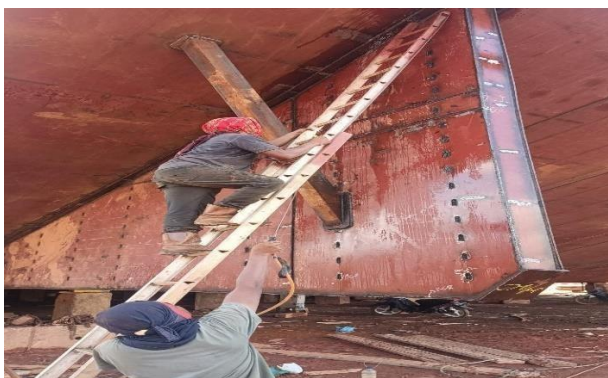
Gambar 2. 41 Proses air pressure test sgeg
