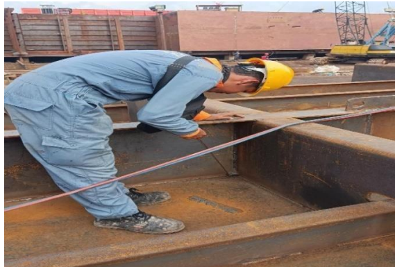
Gambar 2. 24 Inspect welding terhadap Bottom
