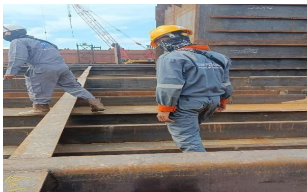
Gambar 2. 2 inspect welding bagian bottom
