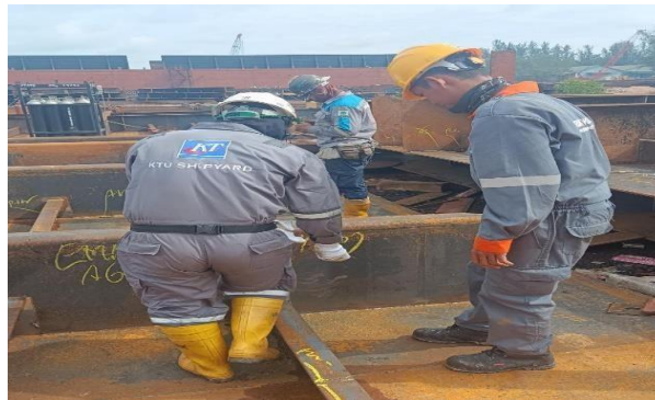
Gambar 2. 10 Inspect welding terhadap main deck
