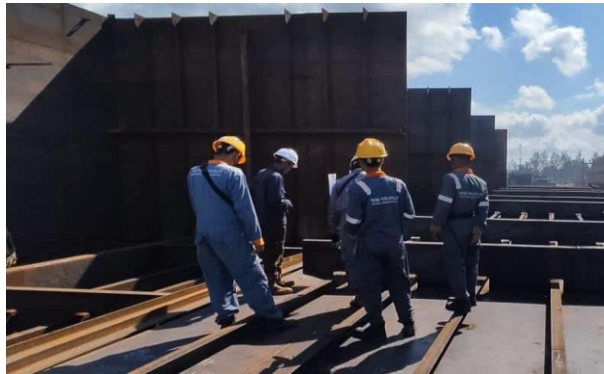
Gambar 2. 15 Inspect welding terhadap longitudinal bulkhead & Bottom
