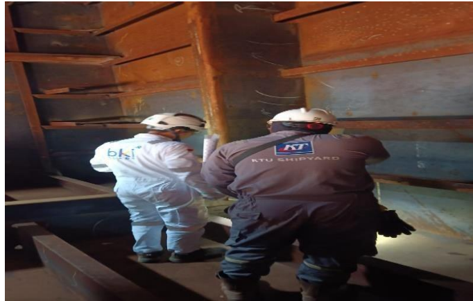
Gambar 2. 33 inspect welding Bersama Surveyor class BKI
