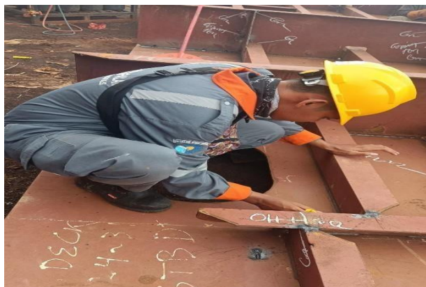
Gambar 2. 1 Proses inspect welding
