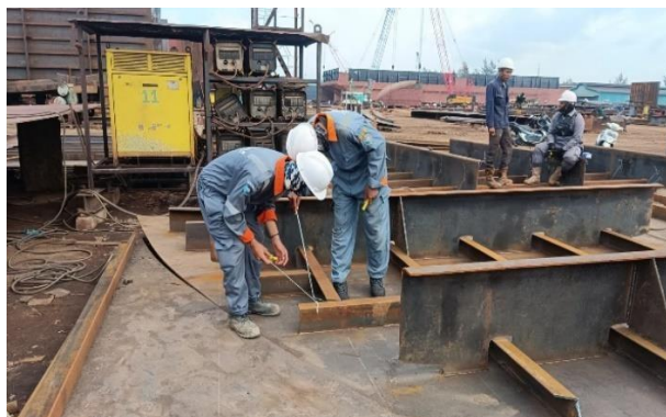
Gambar 2. 66 Inspect welding terhadap longitudinal bulkhead .
