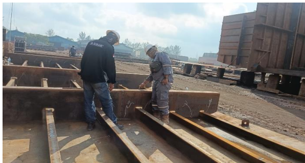
Gambar 2. 54 Inspect welding terhadap side shell
