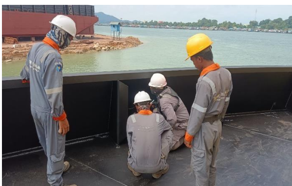
Gambar 2. 67 inspect welding terhadap bulwark
