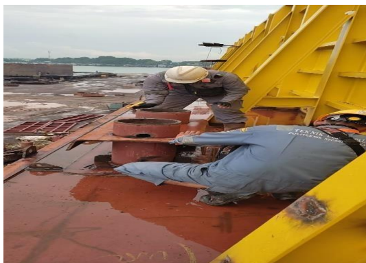
Gambar 2. 6 Inspect welding terhadap Bollard
