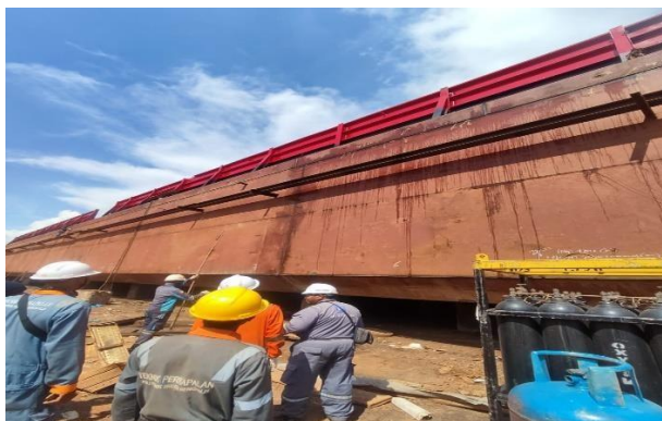
Gambar 2. 40 Proses air pressure test
