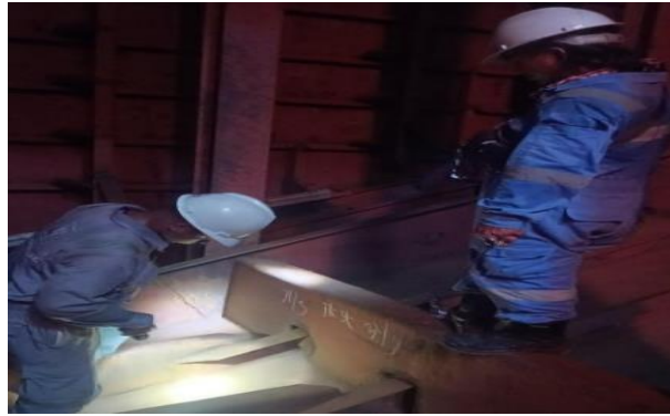
Gambar 2. 25 Inspect welding tangki kapal tongkang
