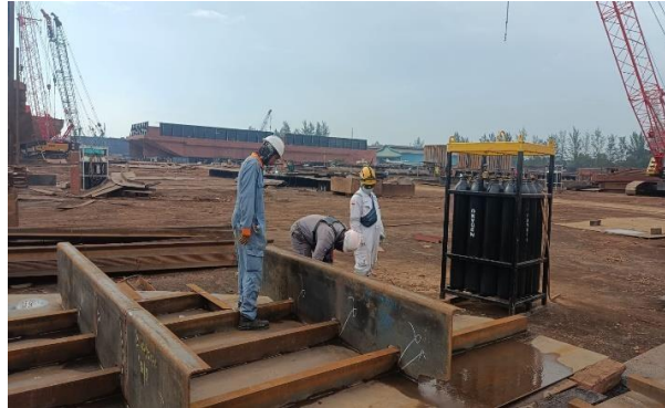
Gambar 2. 68 Inspect welding bersama owner
