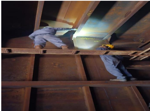
Gambar 2. 26 inspect welding di tangki
