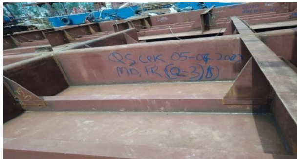
Gambar 2. 5 Inspect welding terhadap main deck
