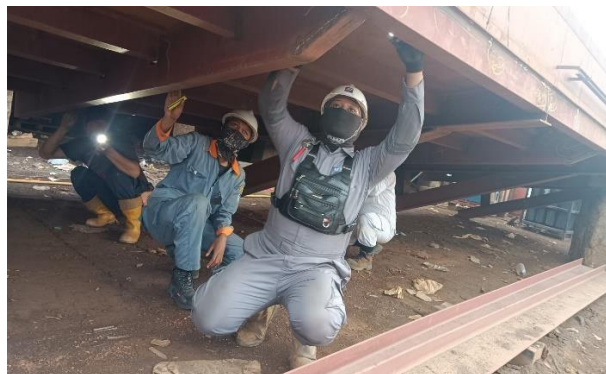
Gambar 2. 69 Inspect welding terhadap side boad
