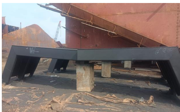
Gambar 2. 32 inspect welding Busher Box
