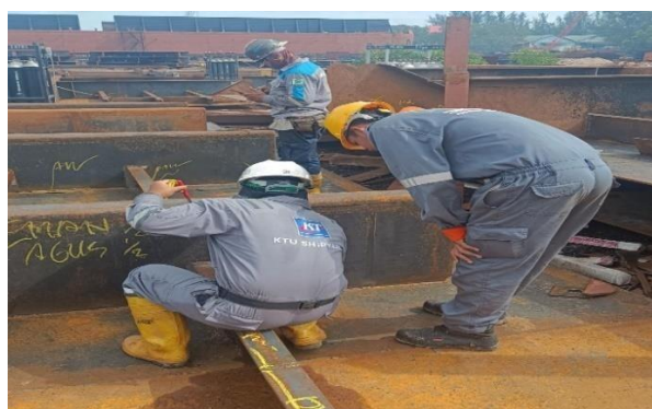
Gambar 2. 12 Inspect welding terhadap Main deck
