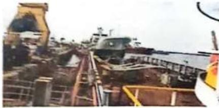
Gambar 1.2 Proses Erection Kapal AHTS
