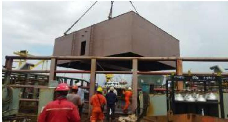
**Gambar 2.26 Proses Erection Slop Tank Pada Main Deck Kapal AHTS**
