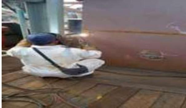
**Gambar2.39 Proses Touch UP Welding**
