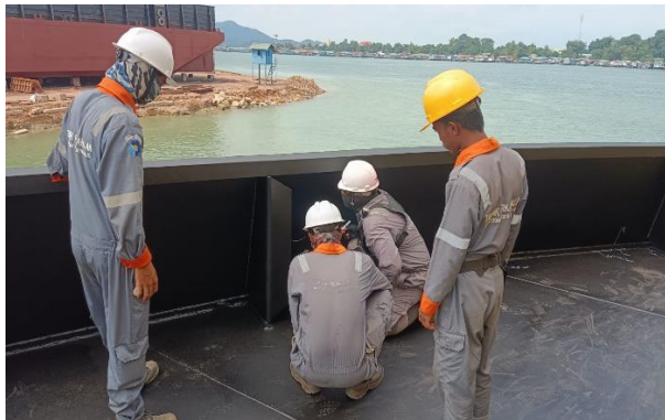
Gambar 2. 57 inspect welding terhadap bulwark.
