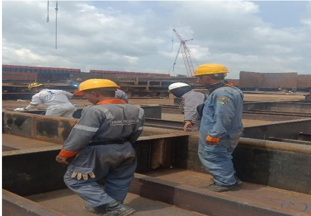
Gambar 2. 28 inspec welding Bersama Owner
