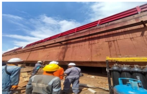
Gambar 2. 38 Proses Air Pressure Test eksternal.
