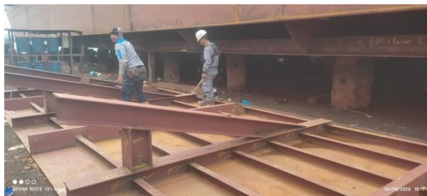
Gambar 2. 54 Inspect welding side board
