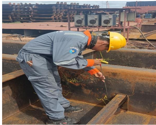
Gambar 2. 18 Inspect welding terhadap main deck
