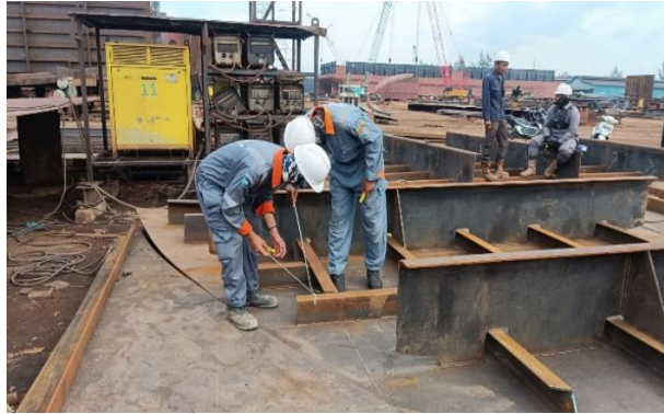
Gambar 2. 56 inspect welding terhadap longitudinal bulkhead.
