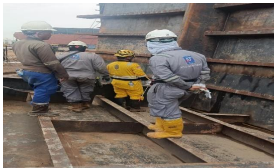
Gambar 2. 20 inspec welding Bersama Owner.
