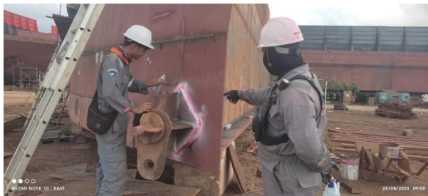
Gambar 2. 55 Proses penetrant test
