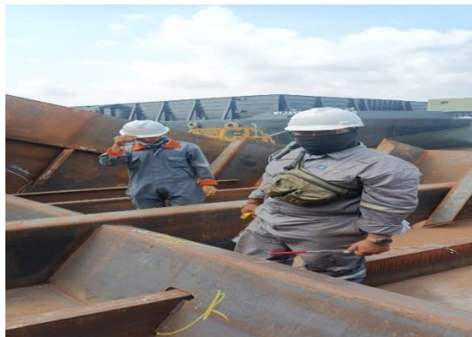
Gambar 2. 43 inspect welding terhadap Bottom
