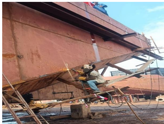
Gambar 2. 19 proses gouging.
