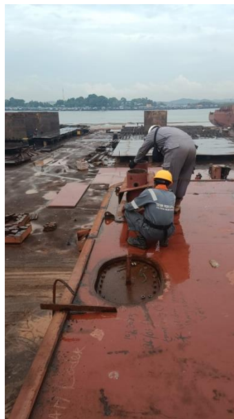
Gambar 2. 6 Inspect welding terhadap Bollard
