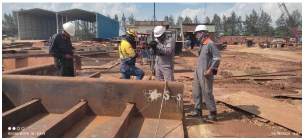
Gambar 2. 52 Inspect welding main deck
