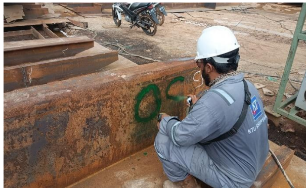
Gambar 2. 50 Proses penandaan panel main deck
