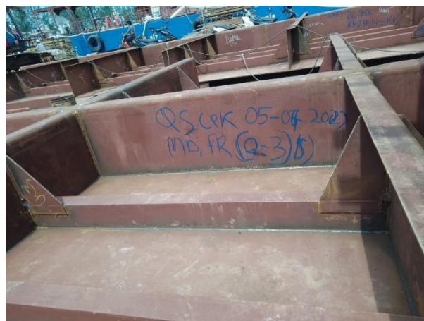
Gambar 2. 5 Inspect welding terhadap Main deck.
