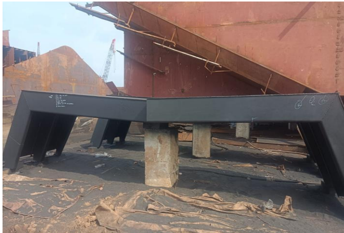
Gambar 2. 31 inspect welding Busher Box
