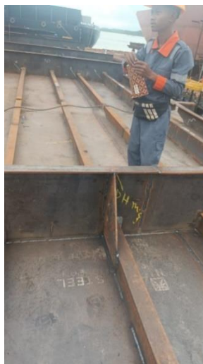
Gambar 2. 11 Inspect welding di Main deck kapal Tongkang.
