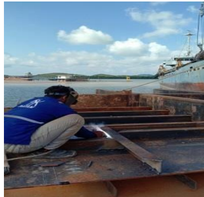
Gambar 1. 40 visual inspect main deck hull 14
