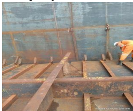
Gambar 1. 33 visual inspect trans bulkhead
