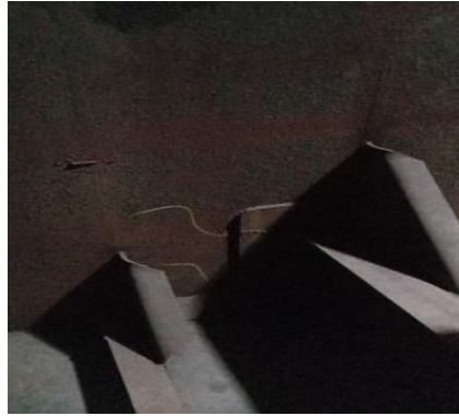
Gambar 1. 34 hasil inspect tangki minus kebocoran
