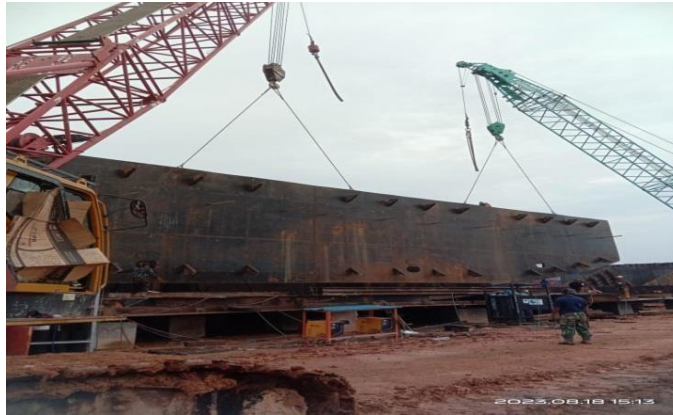
Gambar 1. 57 long bulkhead center port
