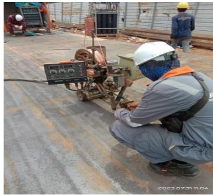
Gambar 1. 36 mencoba mesin SAW
