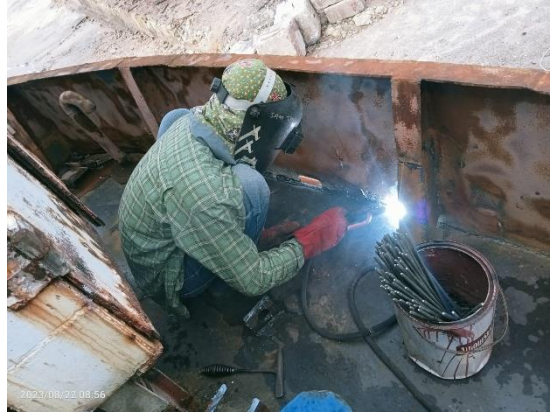
GAMBAR 2. 12 welding alas bulwark
