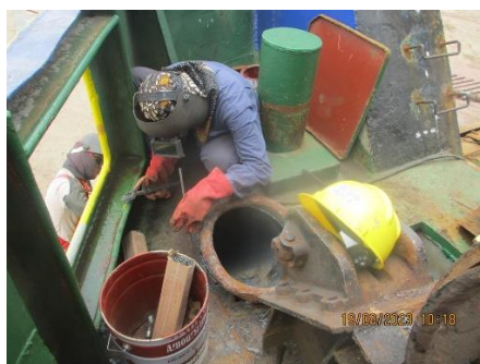
GAMBAR 2. 31 pemasangan pipa urlap jangkar
