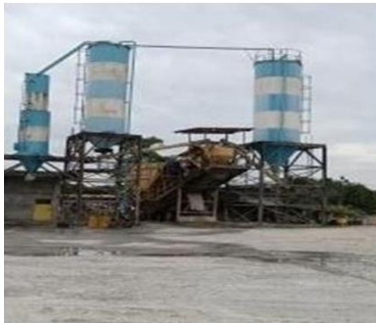
Gambar 1. 7 Mesin Batching Plant
