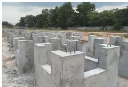
Gambar 2. 2 precast pile cop
