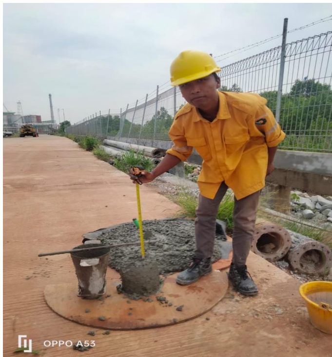
Gambar 3. 8 Uji slump test
