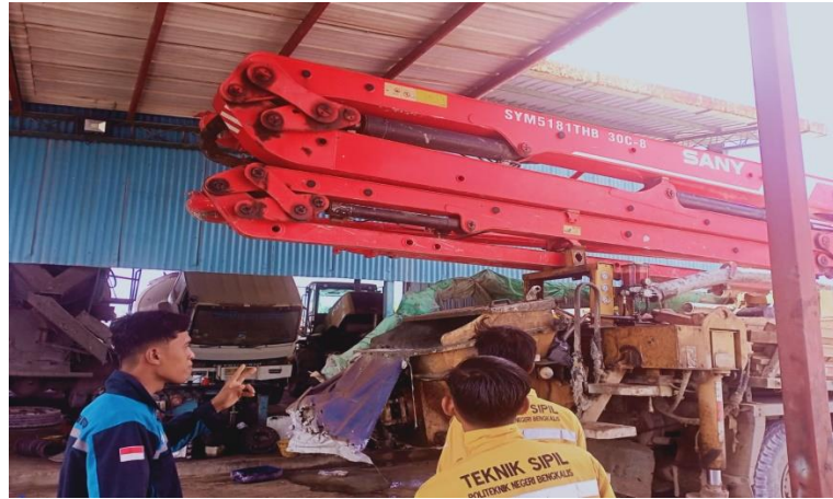
Gambar 3. 1 Alat berat (concrete pump)
