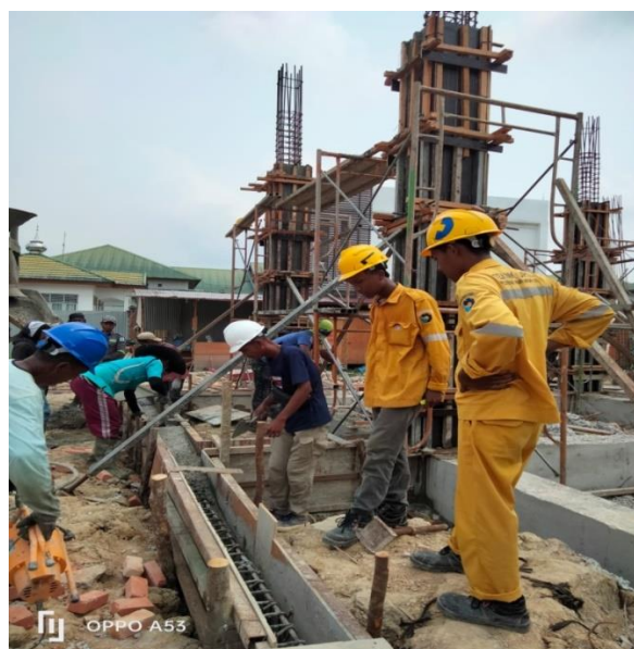
Gambar 3. 24 Pengecoran tea beam
