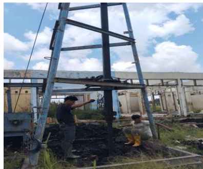
Gambar 3. 13 Pengeboran Bore Pole
