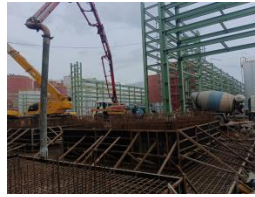
Gambar 3. 47 concrete pump (Sumber : Dokumantasi Proyek, 2023)
