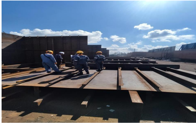
Gambar 2. 17 proses inspect welding longitudinal
