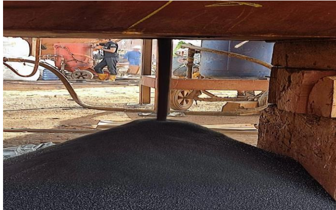
Gambar 2. 11 sandblasting di bagian frash water tug boat
