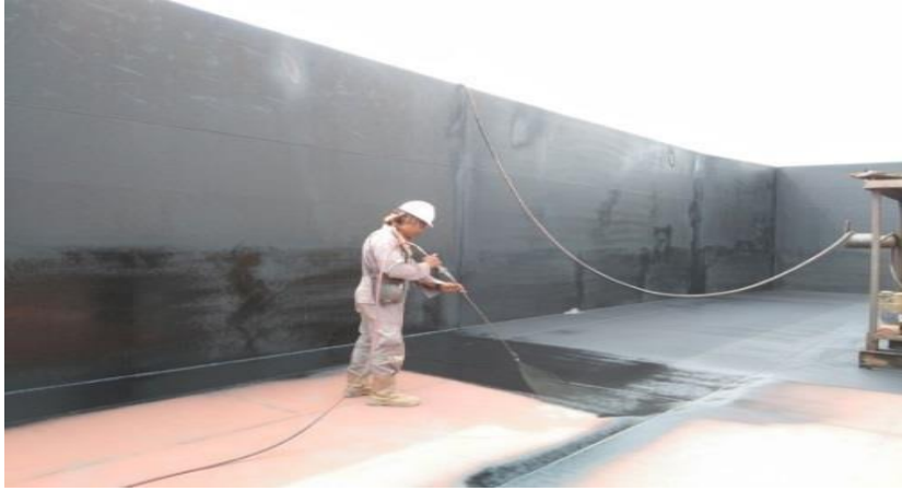
Gambar 2.57 Pengecatan external dack
