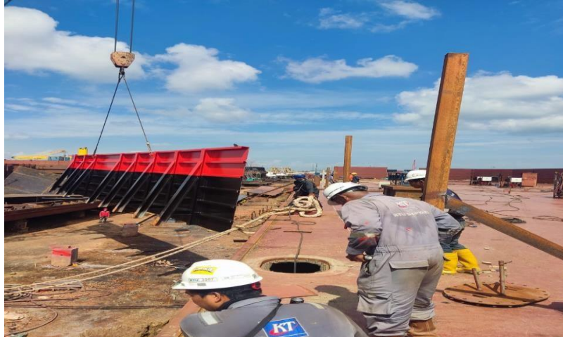
Gambar 2. 21 proses pemasangan sead boat
