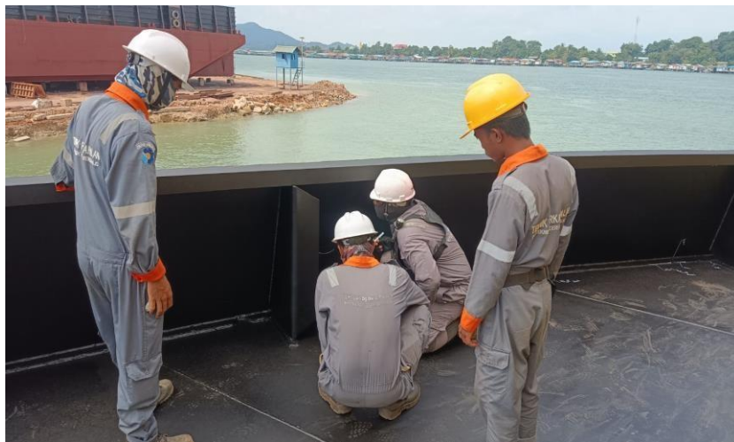
Gambar 2.60 final inspection bulkwork
