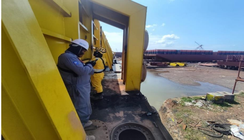
Gambar 2.58 finis inspection tengki
