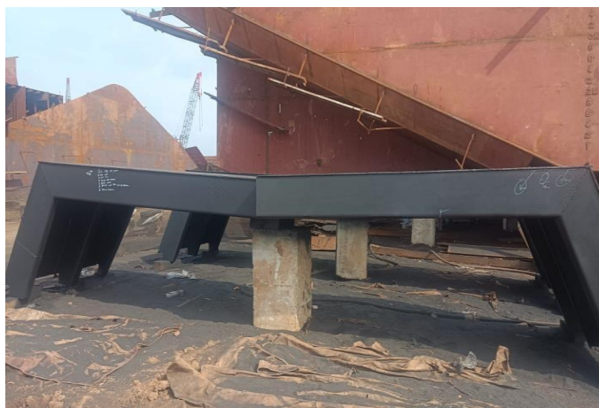
Gambar 2. 38 inspect welding Busher Box
