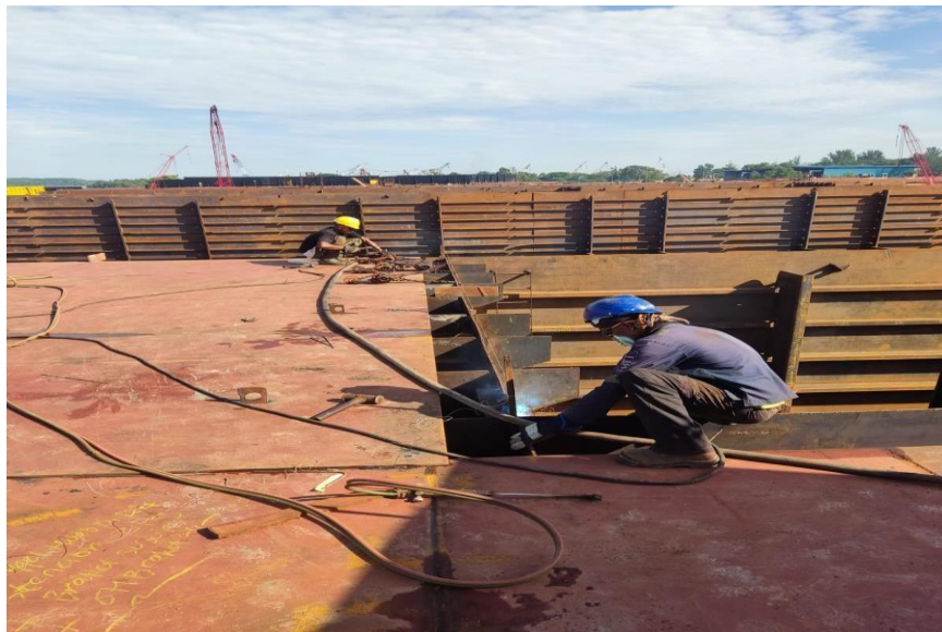
Gambar 2. 35 proses pemasangan panel maen dack
