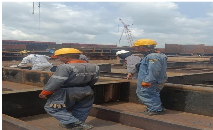
Gambar 2. 36 inspec welding Bersama Owner
