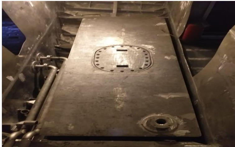
Gambar 2.1 Sewage Threatment Plant
