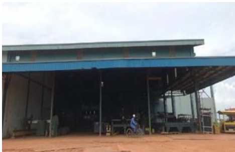
Gambar 1. 3 workshop cutting, bending & rolling
