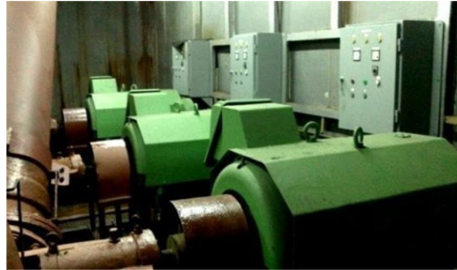
Gambar 1.2 Pompa Graving Dock
