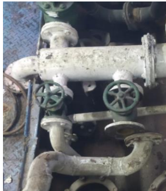
Gambar 3.8 Manifold KM Dharma Ferry II
