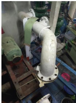
Gambar 3.4 Pipa Ballast Tank KM Dharma Ferry II Sumber :Dokumentasi
