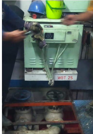
Gambar 3.3 Water Ballast Tank SB KM Dharma Ferry II Sumber :Dokumentasi
