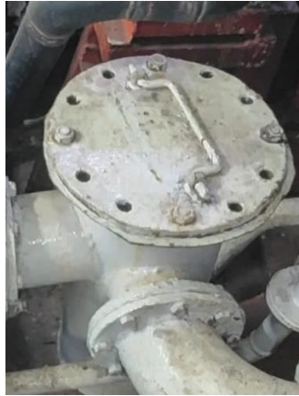
Gambar 3.5 Simplex Strainer KM Dharma Ferry II Sumber :Dokumentasi
