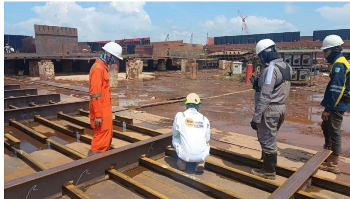
Gambar 2.45 Inspect welding panel longitudinal bulkhead
