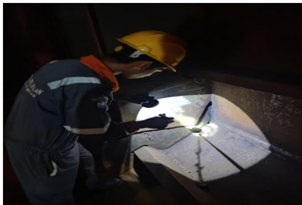
Gambar 2. 21 inspect welding tangki tongkang
