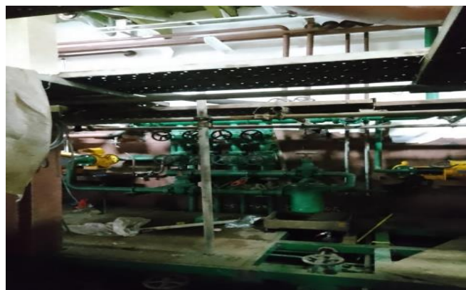
Gambar 2. 32 pipa FO transfer
