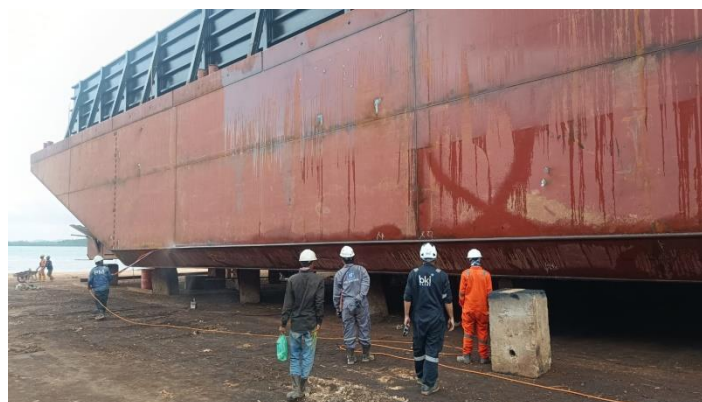
Gambar 2. 56 proses air pressure test eksternal
