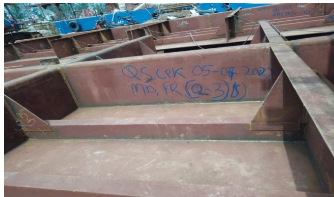
Gambar 2. 5 Inspect welding terhadap main deck
