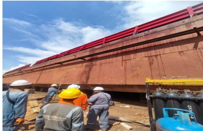
Gambar 2. 34 Proses Air pressure test eksternal
