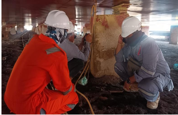
Gambar 2. 43 keel deflection kapal tongkang
