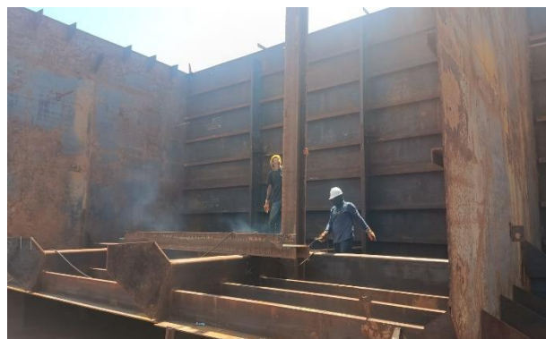
Gambar 2.52 proses pemasangan station
