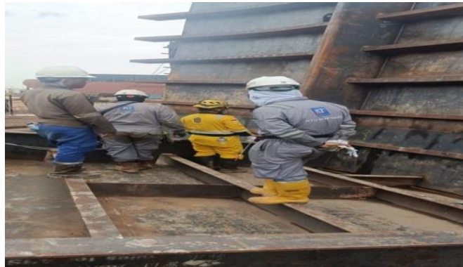
Gambar 2. 17 inspect welding bersama owner
