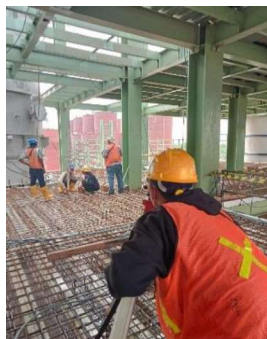
Gambar 3.60 Marking top cor
