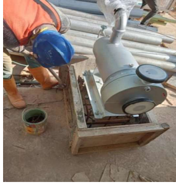
Gambar 3.41 Pemasangan Bekisting Pondasi Equipment
