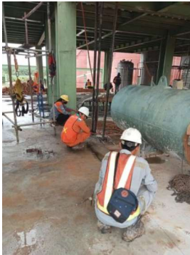
Gambar 3.35 Marking Peletakan Pondasi Equipment
