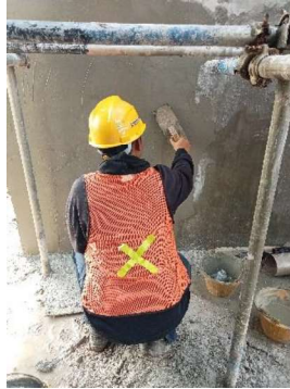
Gambar 3.90 Acian dinding
