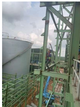
Gambar 3.118 Tiang clading
