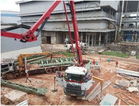
Gambar 3.62 Mobil concrete pump
