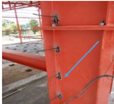
Gambar 3.77 Shear conector
