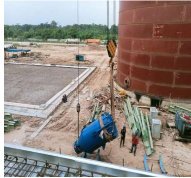
Gambar 3.45 Pengikatan Vessel Tank
