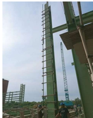
Gambar 3.15 Pemasangan perancah/scaffolding
