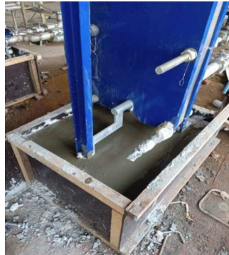
Gambar 3.42 Pengecoran Pondasi Equipment
