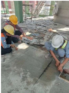
Gambar 3.98 Marking posisi handrail
