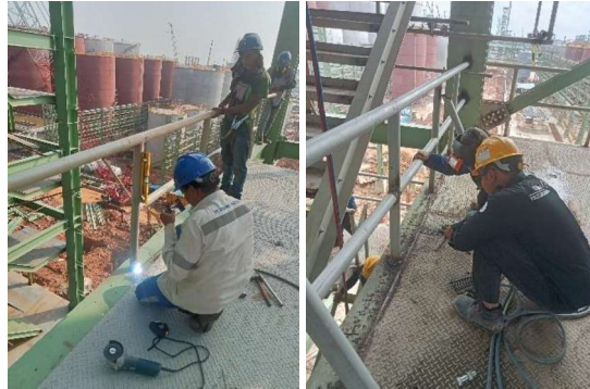
Gambar 3.102 Pengelasan handrail
