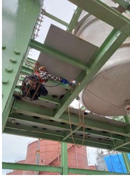
Gambar 3.96 Pengelasan checkered plate
