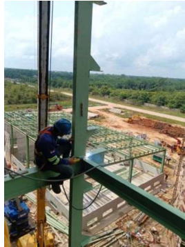
Gambar III.117 Pengelasan clading
