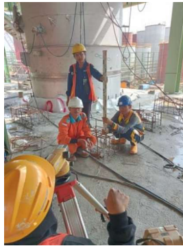
Gambar 3.38 Marking Posisi Angkur Equipment
