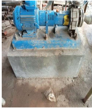
Gambar 3.43 Pondasi Equipment
