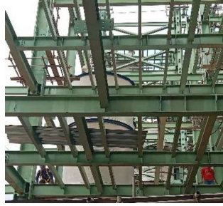
Gambar 3.94 Gording Tumpuan checkered plate
