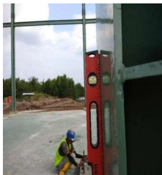
Gambar 3.21 Cek Verticality Kolom.
