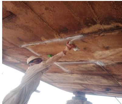
Gambar 2. 61 Penetran Test TB Indopower
