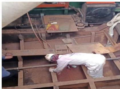
Gambar 2. 62 Penetran Test TB SJP 01
