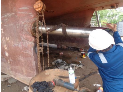
Gambar 3. 15 Pemasangan AS propeller
