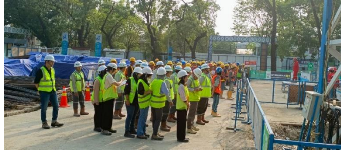
Gambar 3. 32 Safety Morning Talk (Sumber: Dokumentasi Lapangan)
