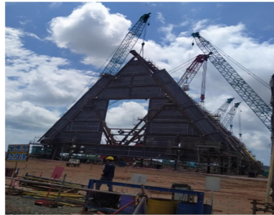
Gambar 2.47 Lifting Jacket Leg A3
