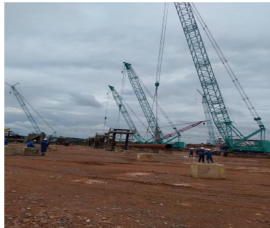
Gambar 2.19 Lifting jacket leg B2
