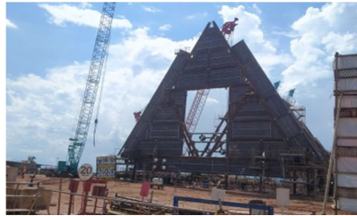
Gambar 2.45 Lifting mudmatet
