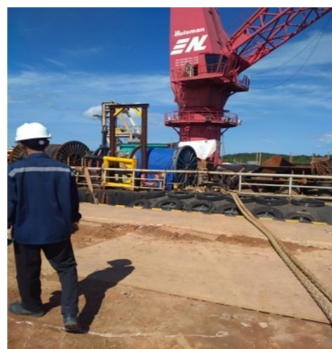
Gambar 2.14 Jetty PT. MEB
