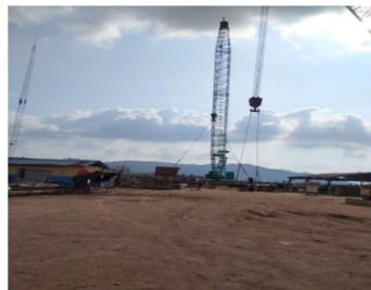
Gambar 2.37 Proses lifting panel Elevasi (-) 23000
