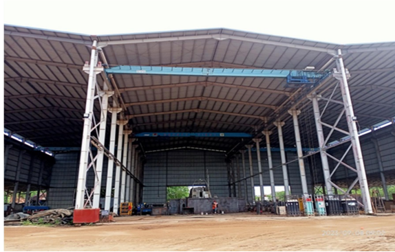
Gambar 1.2 Main Workshop Fabrication
