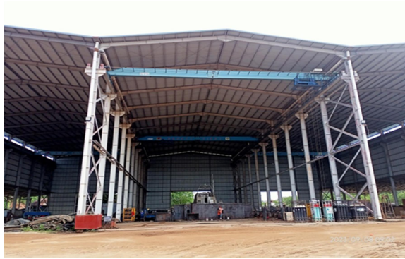
Gambar 1.2 Main Workshop Fabrication
