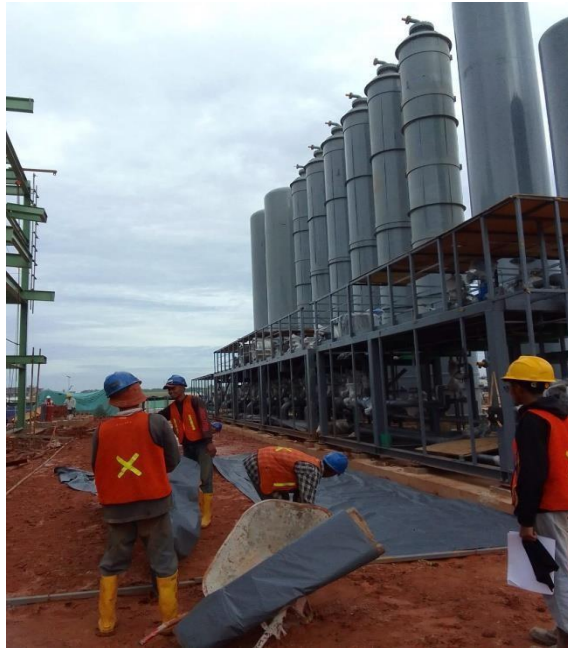
Pekerjaan lc ( lean concrete ) area reformer
