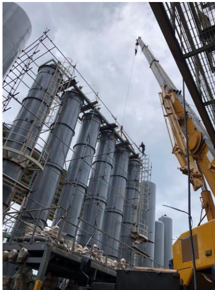
ERECTION HENDRIL AREA PLANT H2 ALIGAS TABUNG
