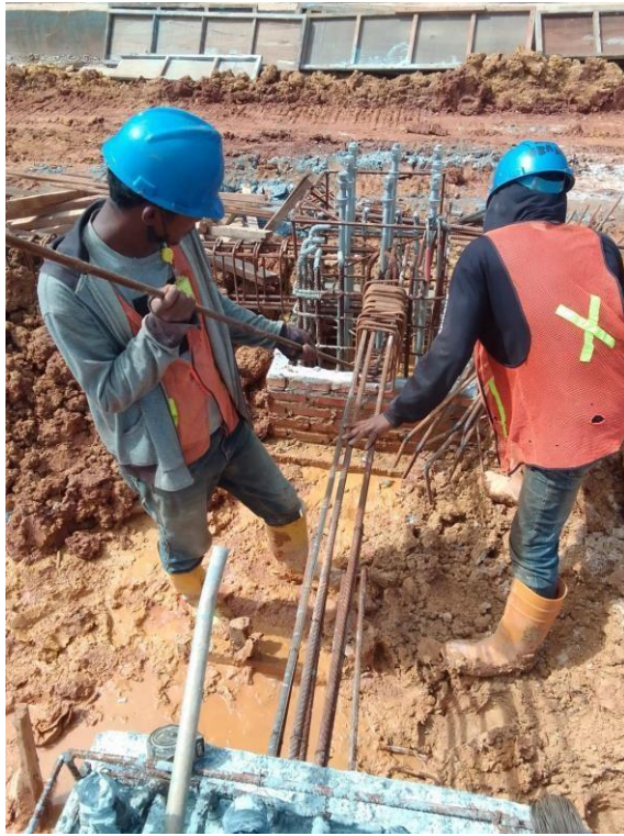
Install ribar piperack internal area compressor
