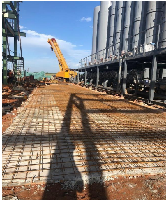
Install tulangan area reformer
