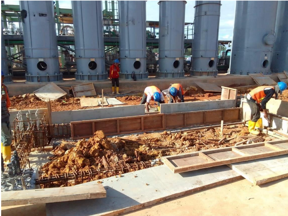
Install Bekesting piperack internal
