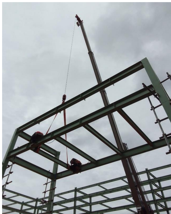
Install balok/beam area reformer
