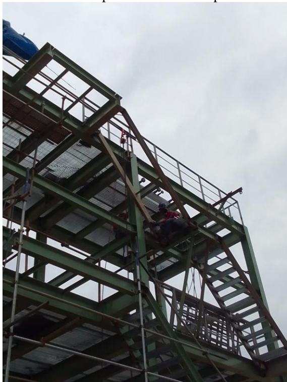
Pengelasan tangga el. 8500 area reformer
