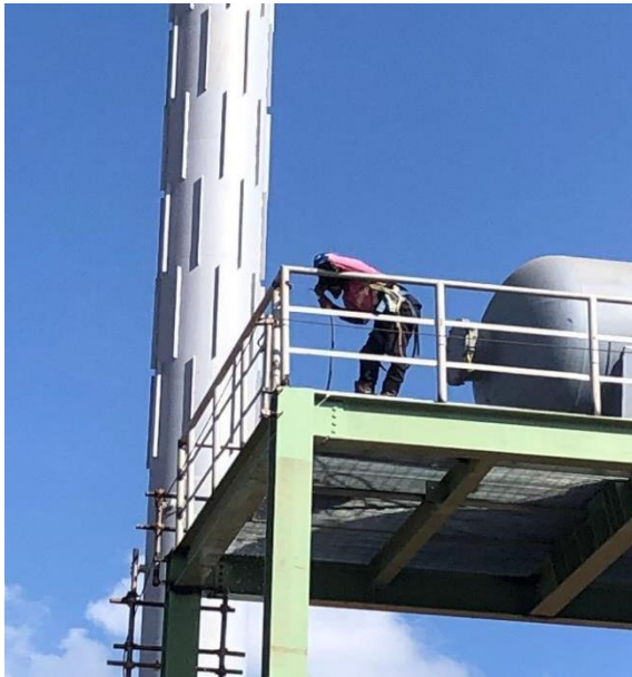
Install grating area reformer
