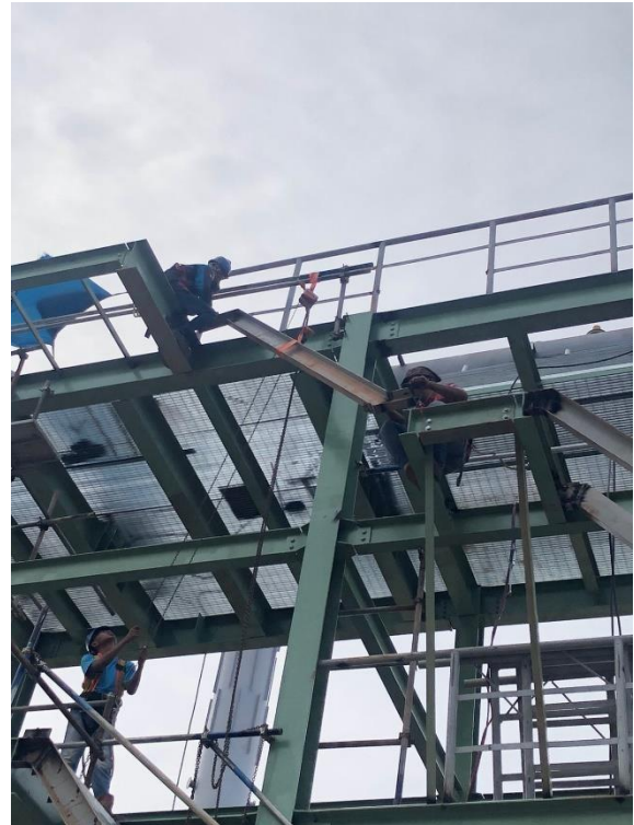
Install tangga el.8500-11000 area reformer
