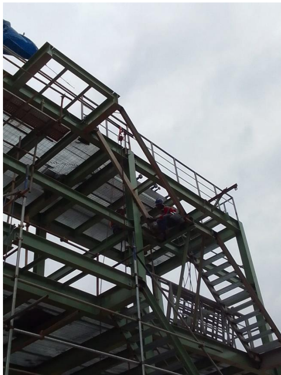
Install tangga el.8500-11.000 area reformer
