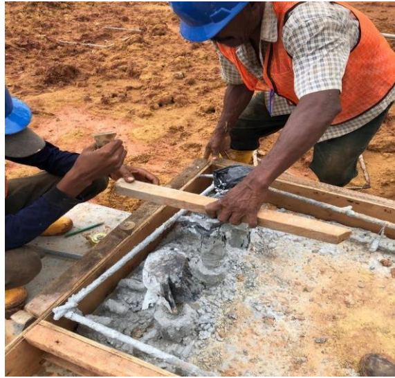
Install pedestal 1300 x 900 area compresor
