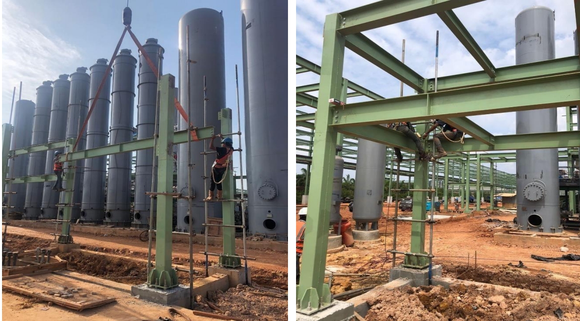
Install balok area compressor el.3000 – 4500
