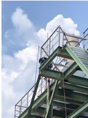
ERECTION KOLOM INSTAN AREA REFORMER
