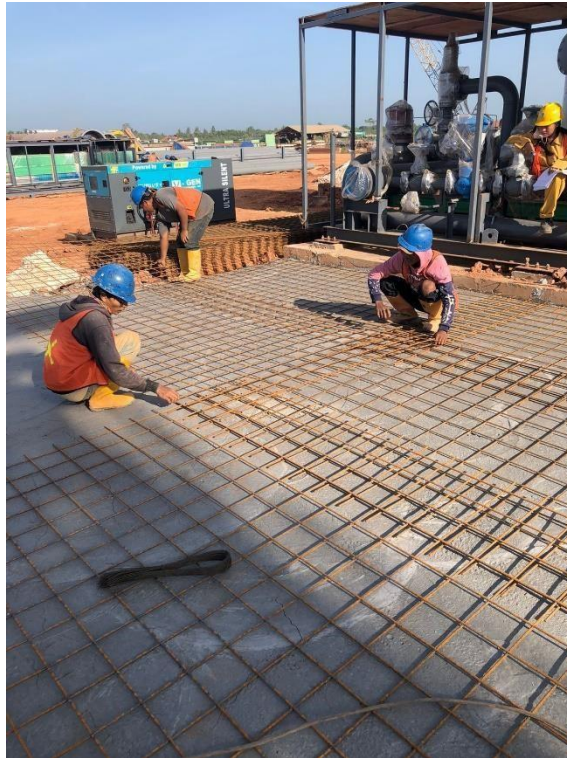
Install tulangan rigid pavement reformer
