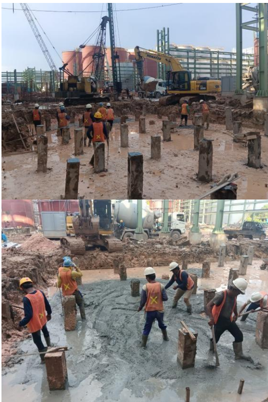
Pengecoran lc colling tower
