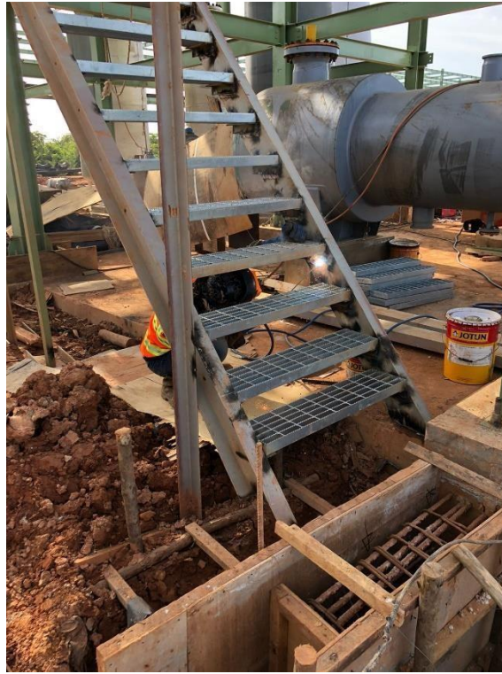
Install tangga area reformer el.3000
