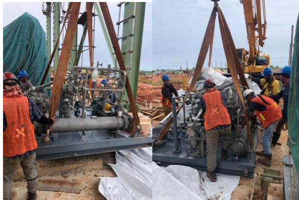
Gambar 3. 24 erection equipment compresor (Sumber : Dokumantasi Pribadi, 2023)
