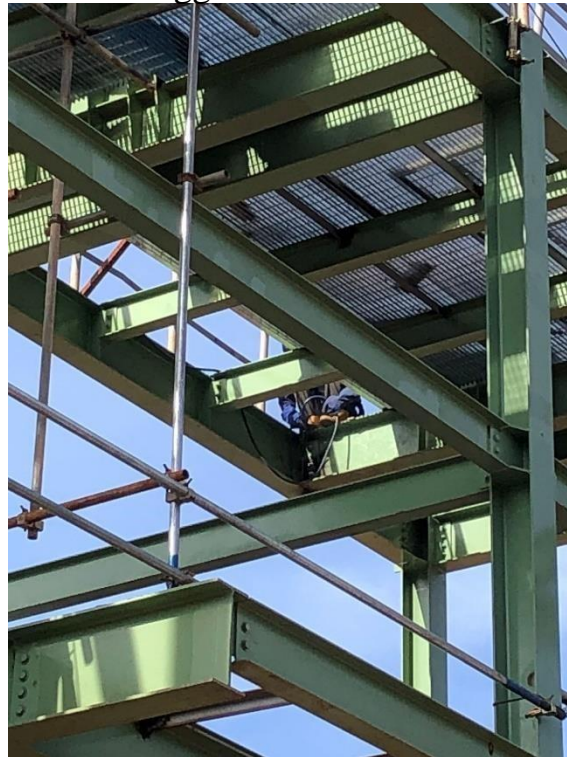
Install grating area reformer el.8500
