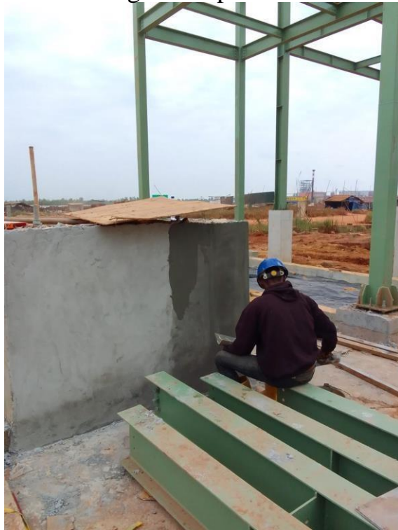
Finishing beton area compresor
