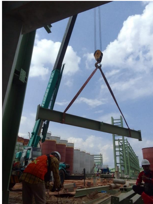
Erection kolom el.23000
