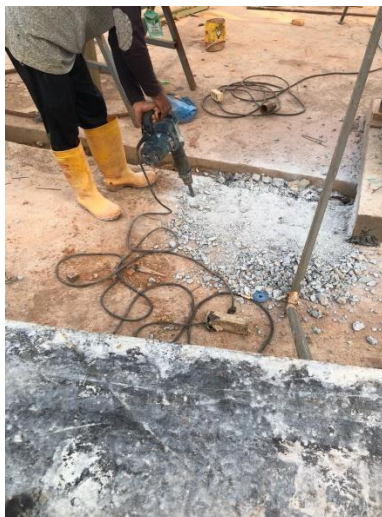
PENBOBOKAN/PERAPIAN PLAT LANTAI AREA PLANT H2 ALIGAS
