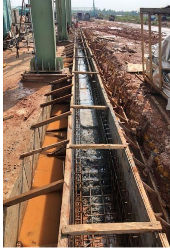
Pengawasan Install Mall Gater
