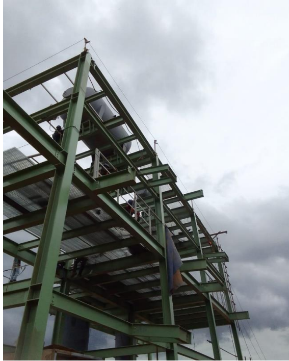
Install grating area reformer
