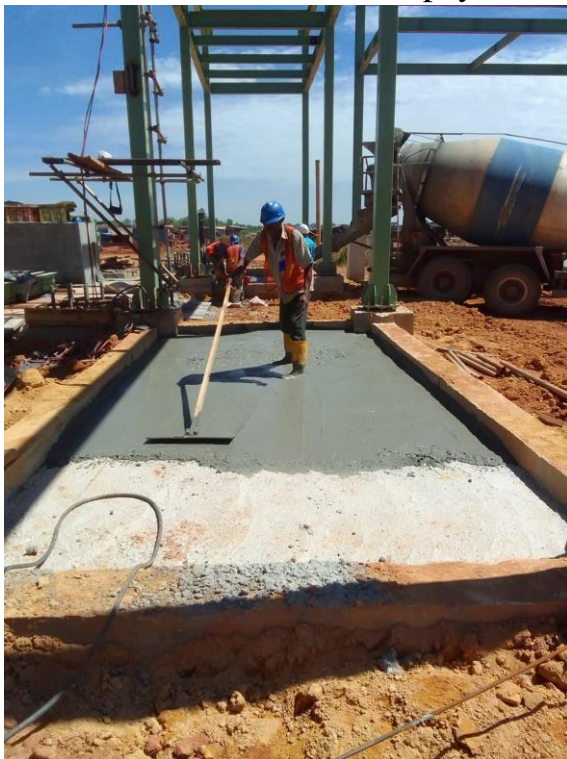
Pengecoran area reformer el.3000
