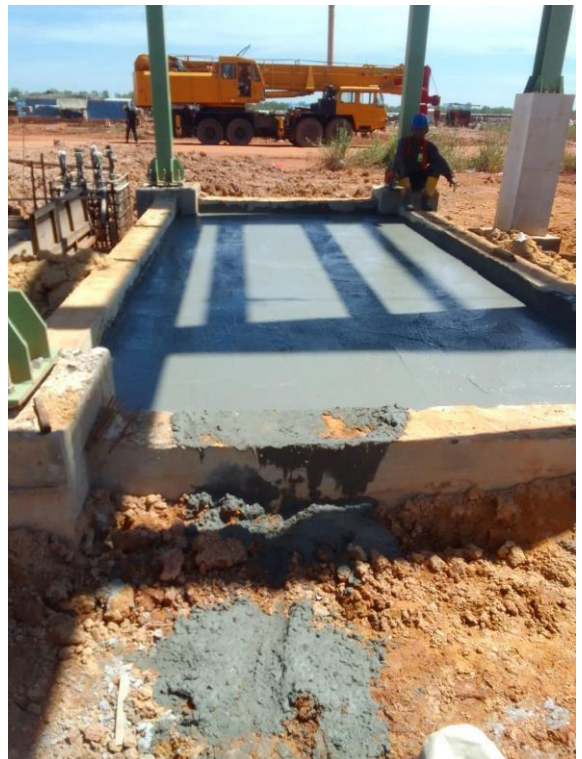
Pengecoran area reformer el.3000
