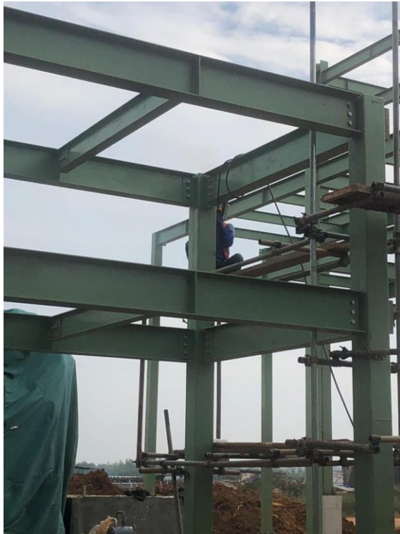
Install balok area compresor
