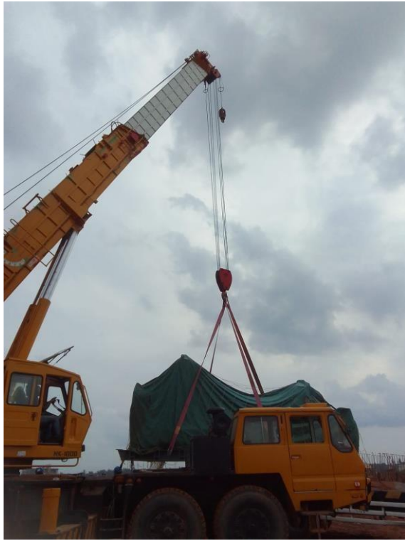
Erection compressor diarea compressor
