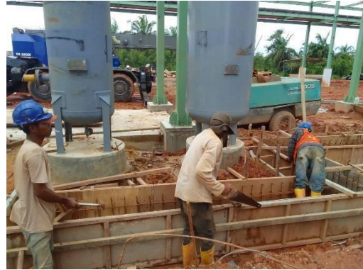
Instal bekesting gater area compressor
