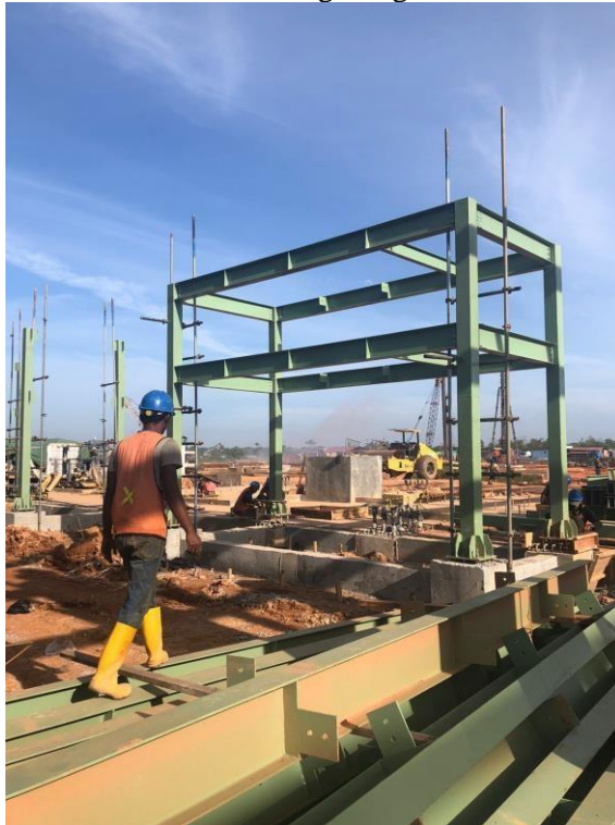
Install struktur area compressor
