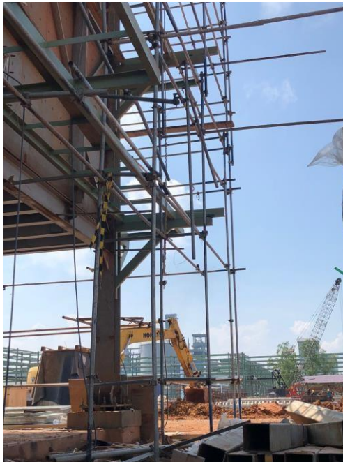
PENGELASAN HENDRIL AREA PLANT H2 ALIGAS
