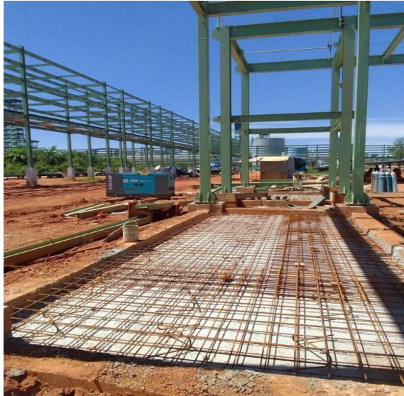
Instal tulangan plat lantai el.3000 area rigid payment reformer
