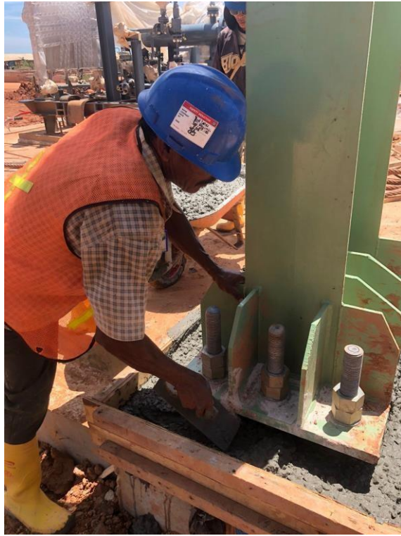
Pengecoran pedestal area compressor
