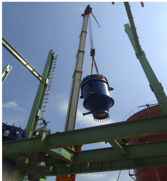
Erection feshel el.14600
