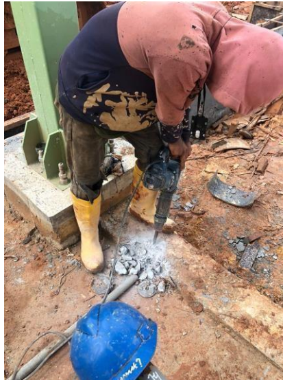
PENBOBOKAN/PERAPIAN PLAT LANTAI AREA PLANT H2 ALIGAS
