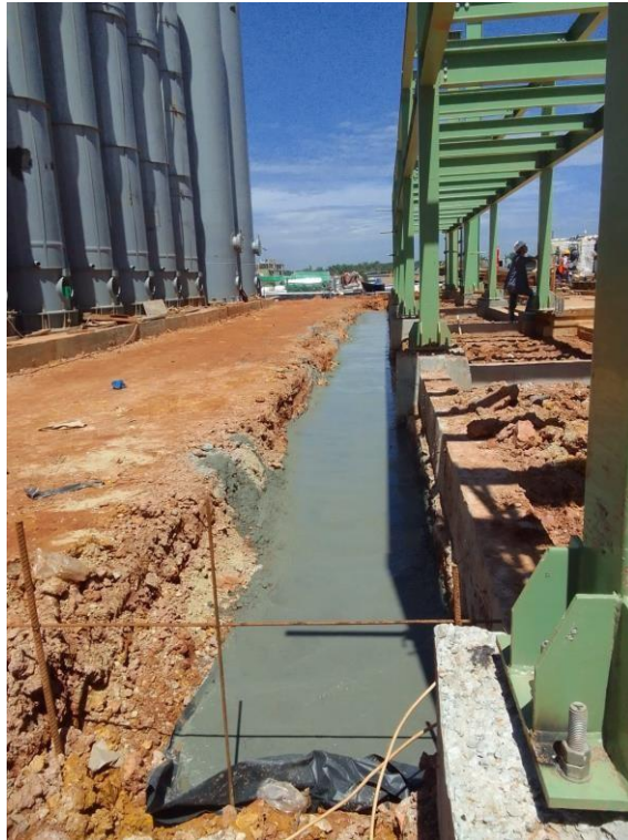
Pengecoran lantai kerja gater area compressor
