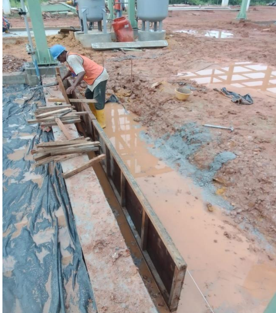
Install bekesting grater area compressor
