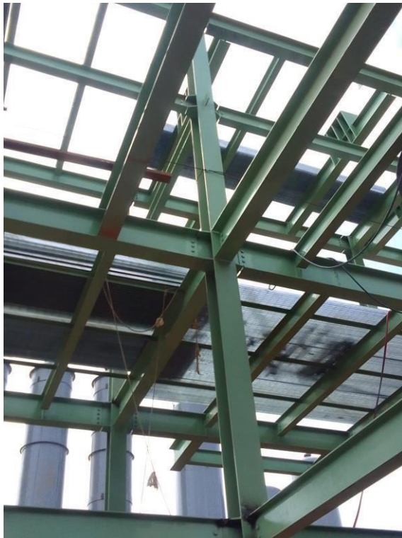
Install grating area reformer
