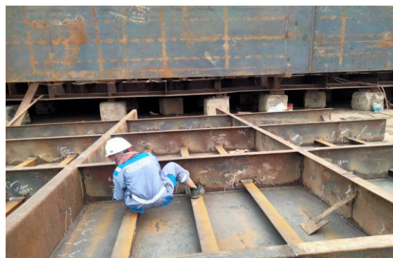
Gambar 2. 24 Welding dibagian Main Deck
