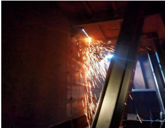
Gambar 2. 47 Cutting bagian tangki
