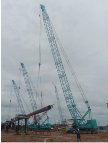
Gambar 2.13 Proses Lifting Jacket
