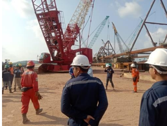
Gambar 2.20 Job Safety Meeting melaksanakan Lifting X-Bracing
