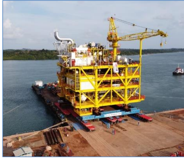
Gambar 3.14 Proses Loadout Topside
