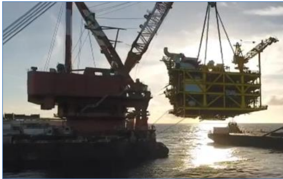
Gambar 3.17 Proses Instalisasi Topside
