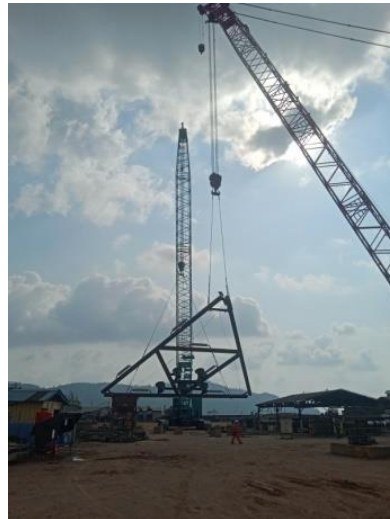
Gambar 2.21 Pengangkatan X-Bracing ( Lifting X-Bracing )
