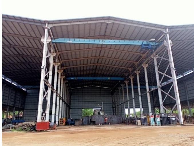
Gambar 1.2 Main Workshop Fabrication
