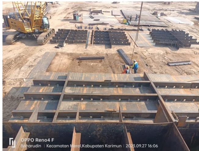
Gambar 3.12. Sub-Block Assembly
