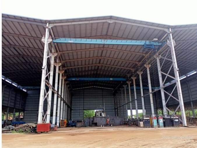
Gambar 1.2 Main Workshop Fabrication
