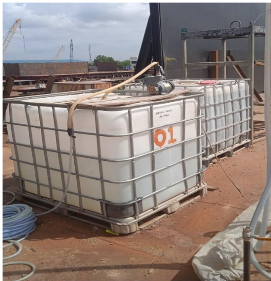
Gambar 6.10 Water tank air test
