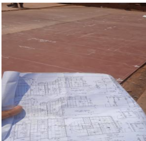
Gambar 5.12 Pengecekan markingan Bridge House
