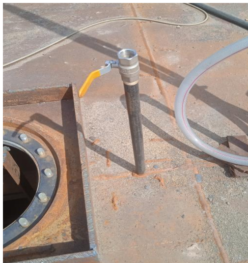
Gambar 6.13 Lubangi samping mainhole
