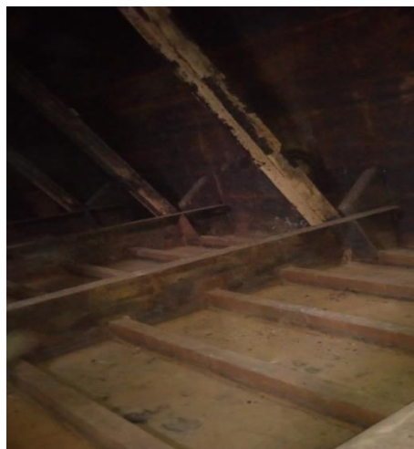
Gambar 2.29 Pengecekan rembesan air
