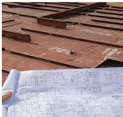
Gambar 5.4 Fit-up Bridge
