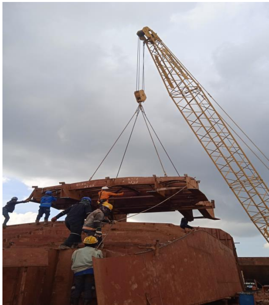
Gambar 5.21 Erection Engine Girder
