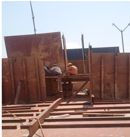
Gambar 5.15 Erection Bridge Deck
