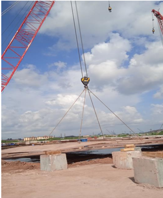
Gambar 3.8 Erection Bottom Hull 025
