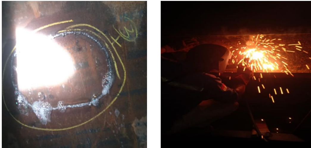
Gambar 6.24 Proses repair kebocoran
