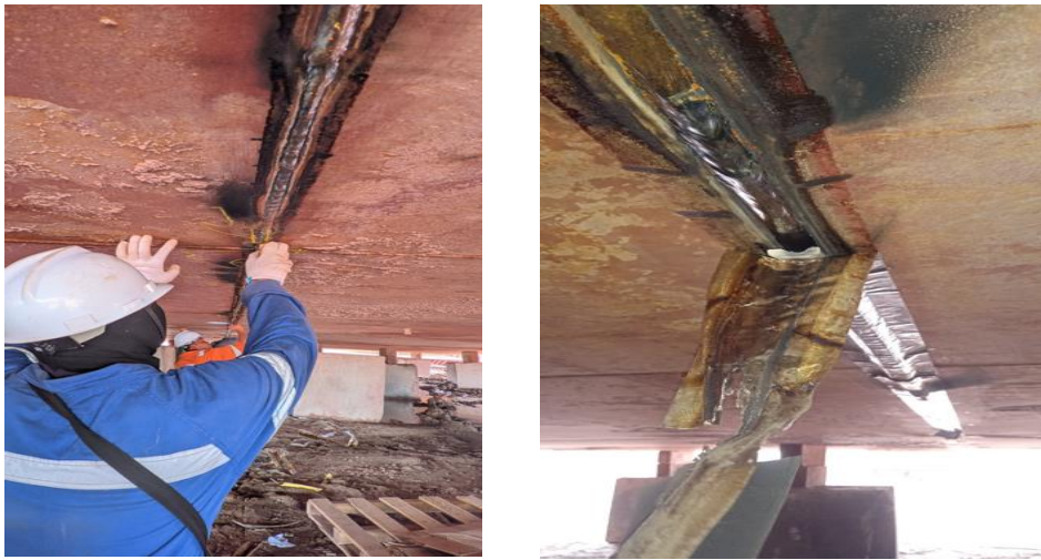
Gambar 4.1 Pengecekan Welding Backing Cramic
